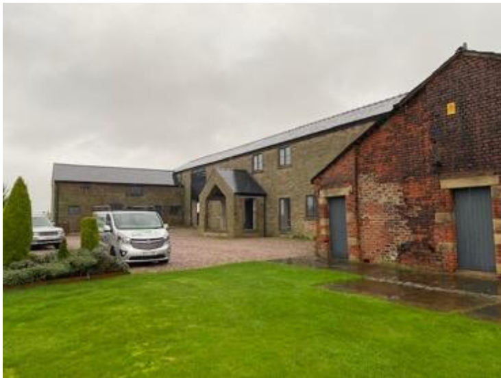
Fig. 1, Former farmyard with outbuildings
