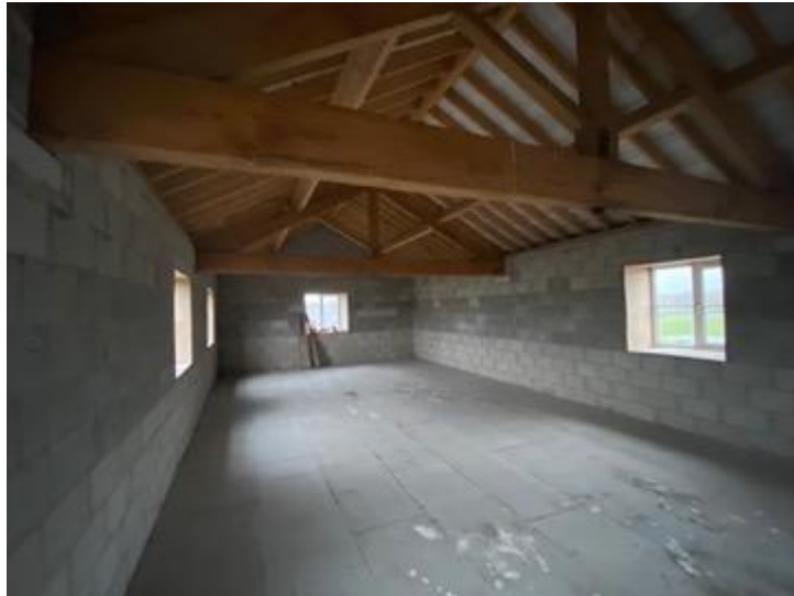
Fig. 12, Internal view FF of Barn
