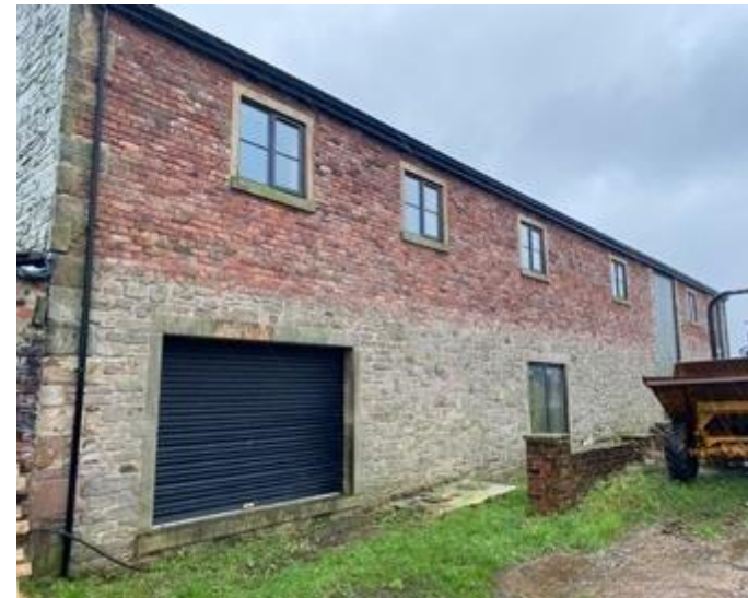
Fig. 10, Rear elevation of barn
