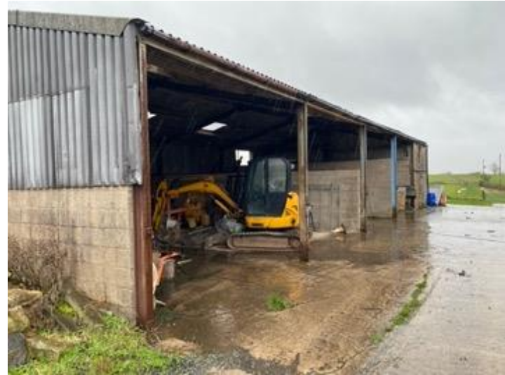
Fig. 17 Open sided barn
