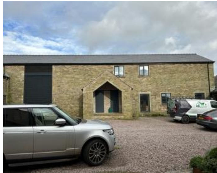
Fig. 9, External view of Barn facing courtyard
