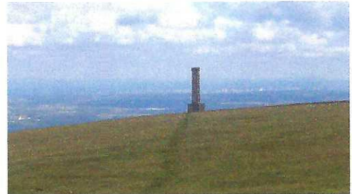
The Peel Monument above Holcombe
