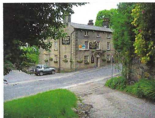
The Shoulder of Mutton public house
