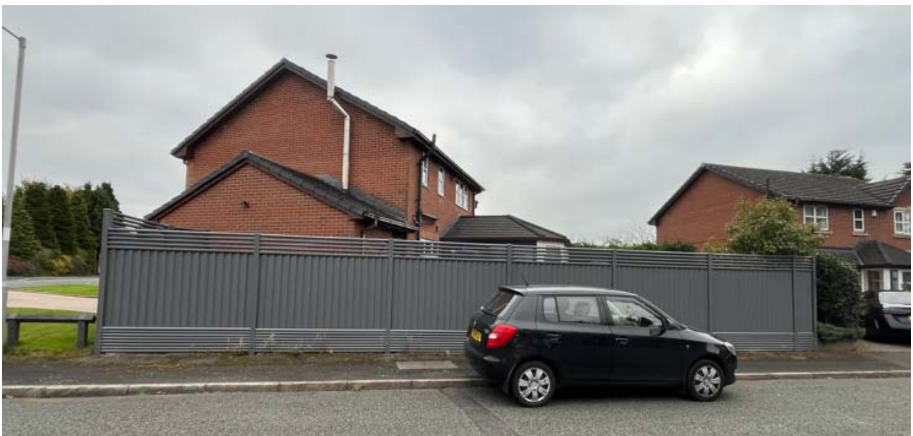
New fence viewed from the side road
