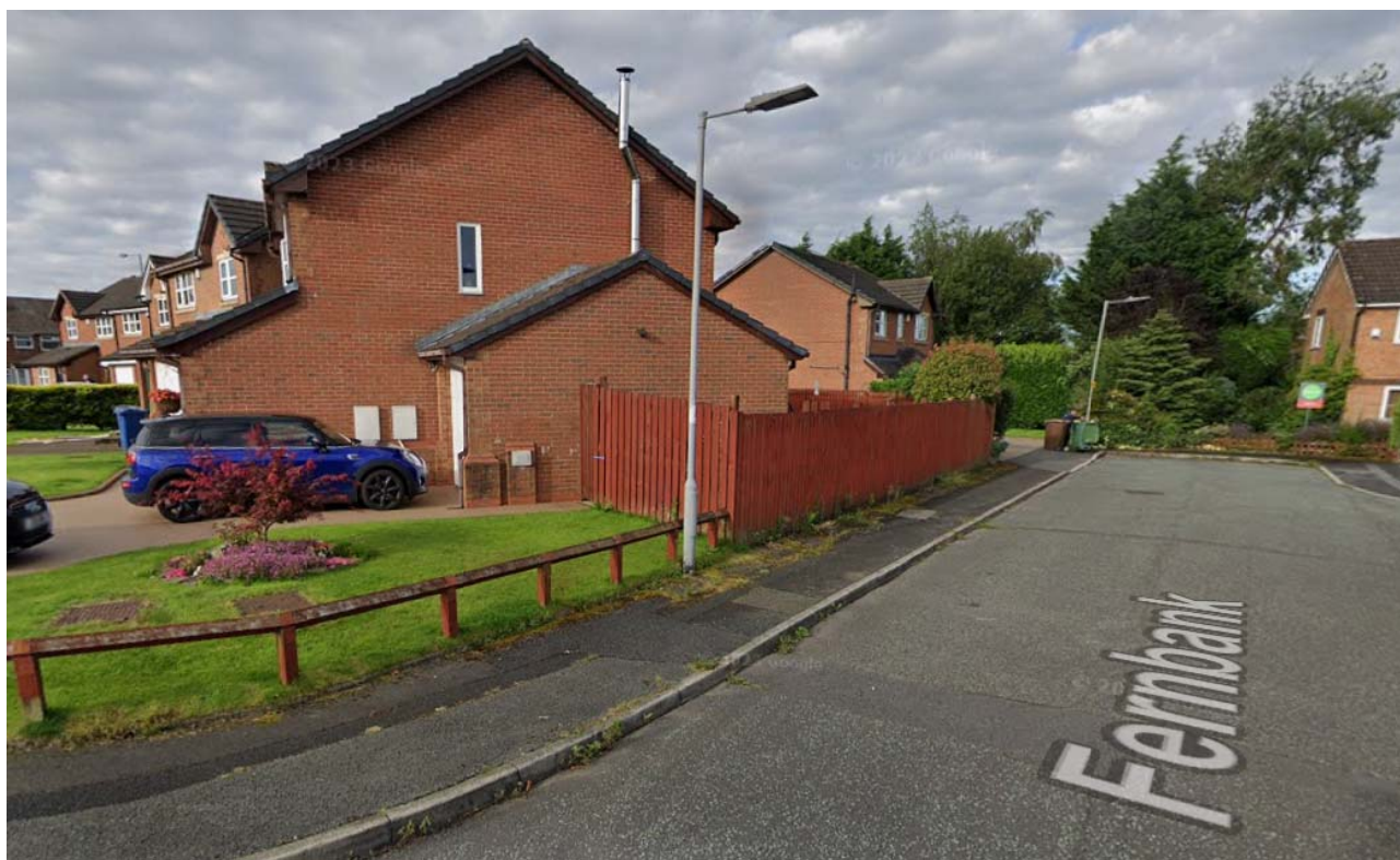
Photos from 2023 showing original timber fence (from Google Streetview)
