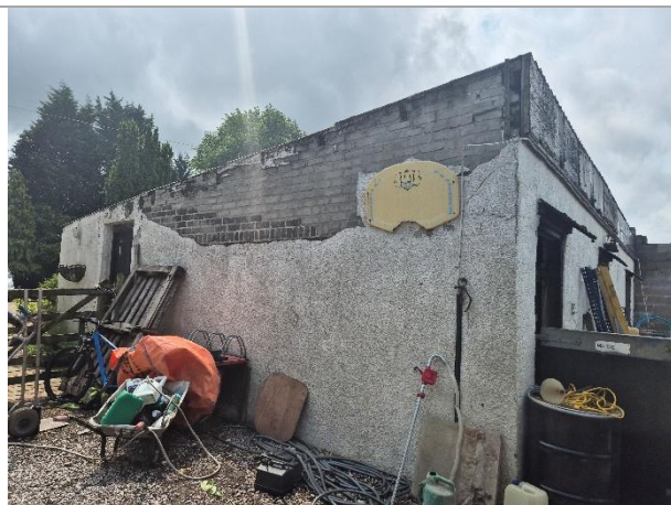
Photo 11: Eastern elevation of the Stable
