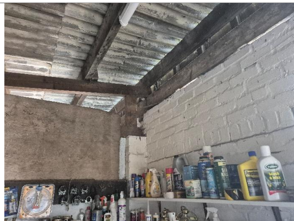
Photo 14: Interior of the Stable
