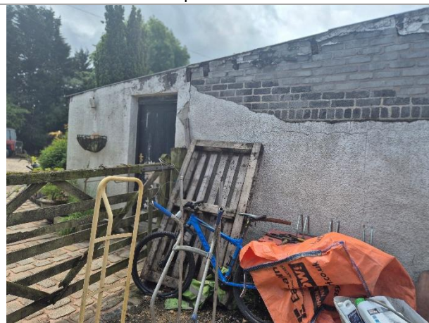
Photo 12: Eastern elevation of the Stable
