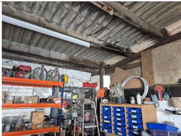
Photo 15: Interior of the Stable
