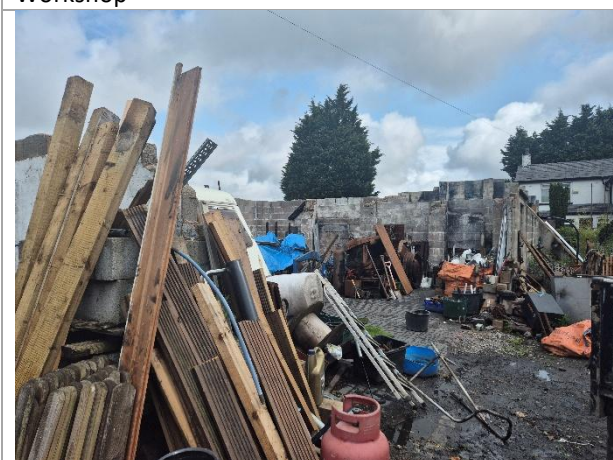
Photo 3: Hardstanding with debris
