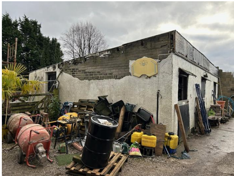
Image 6 – Attached storage building
