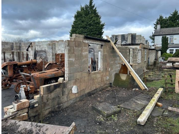
Image 5 – Rear elevation of barn
