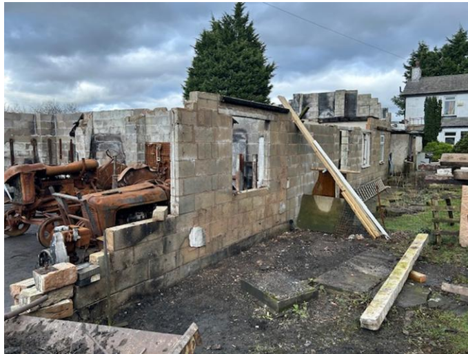
Image 4 – Rear elevation of barn
