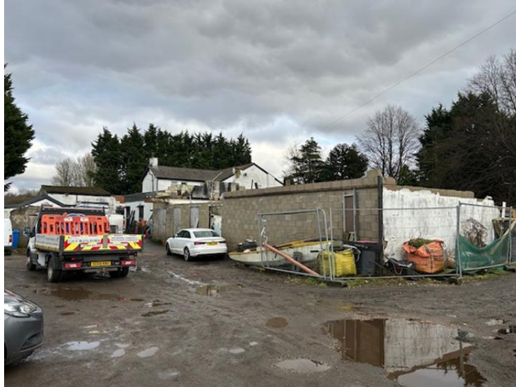
Image 2 - Existing barn and storage buildings
