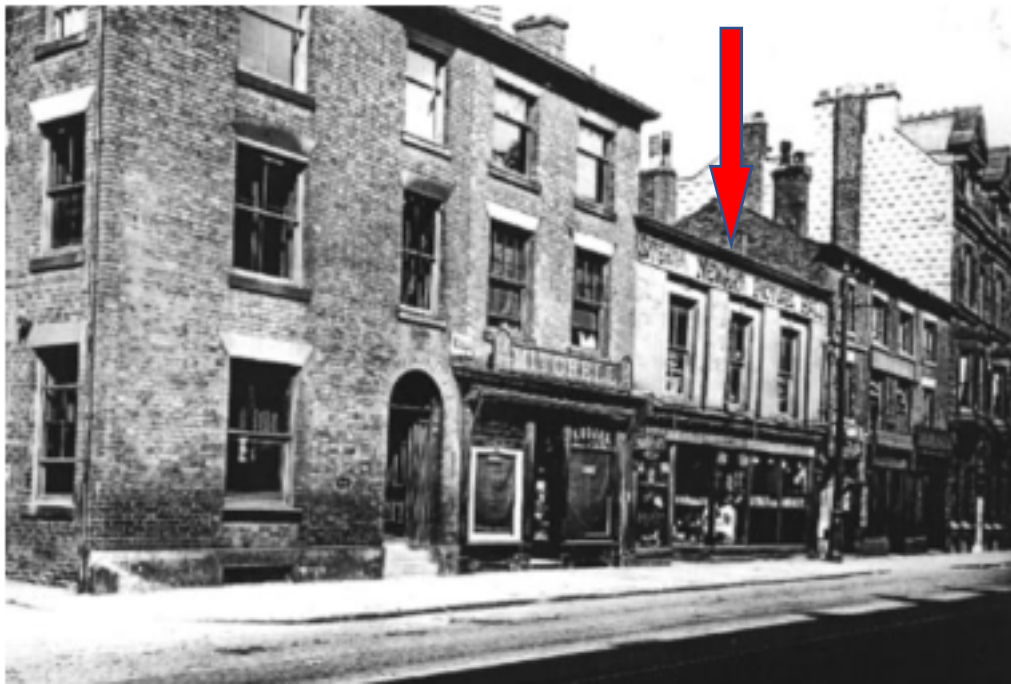
Image of application site: 12 Bolton St.
