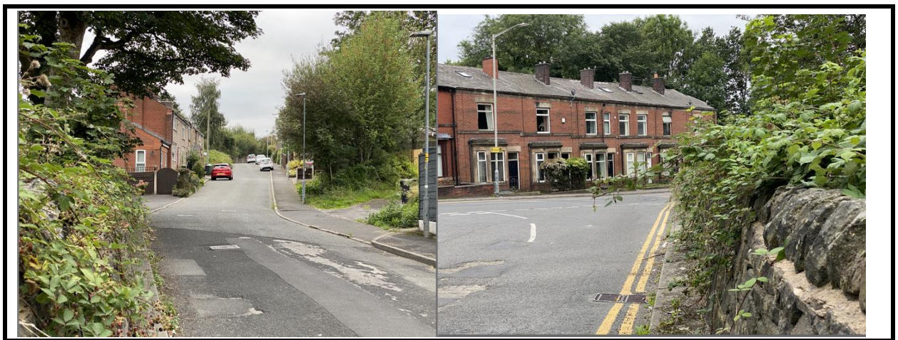
View left and right from Woodgate Hill Road site access
