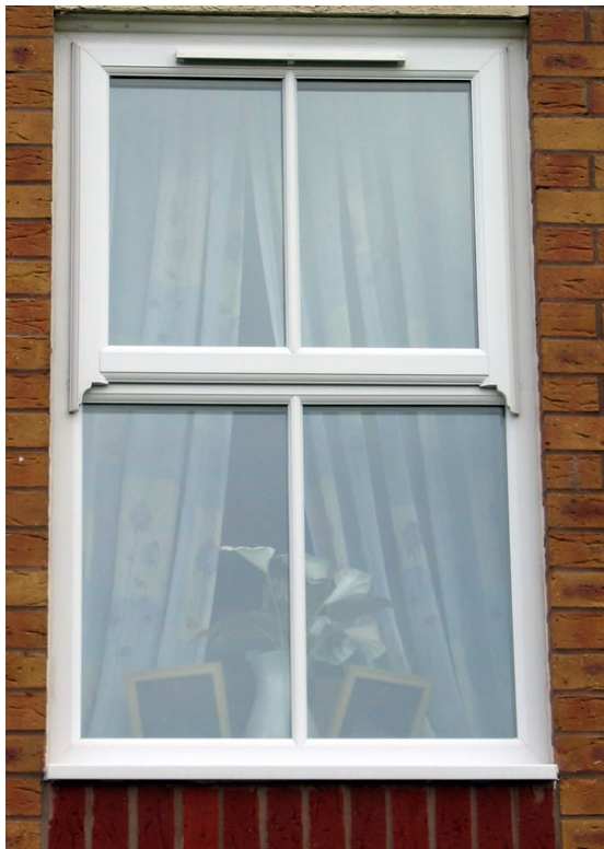
Figure 4: 70mm mock sash window frame from proposed manufacturer (note the proposed windows would not include the central vertical bar shown in this illustration)
