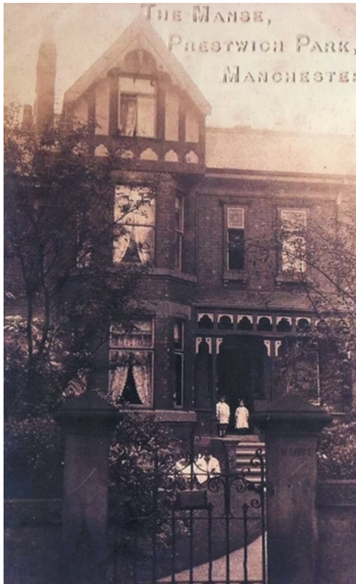
Figure 7: front elevation of no.36 soon after construction showing a mixture of window types, notably casement windows to the ground floor and sash windows to the first floor of the bay (photograph believed to be the turn of the 19 th /20 th century i.e. within 5 years of construction).
