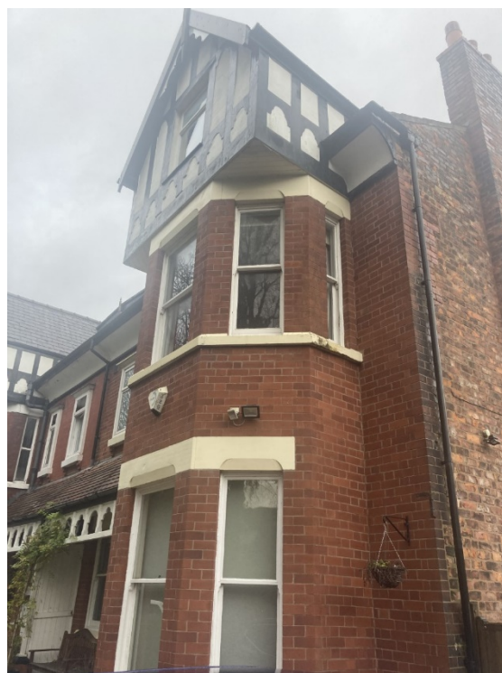
Figure 1b: side of bay showing small side windows to first floor bay.
