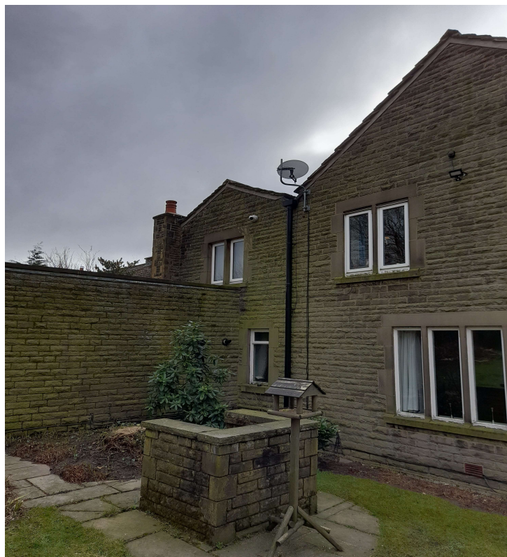
View of site/northern elevation.
