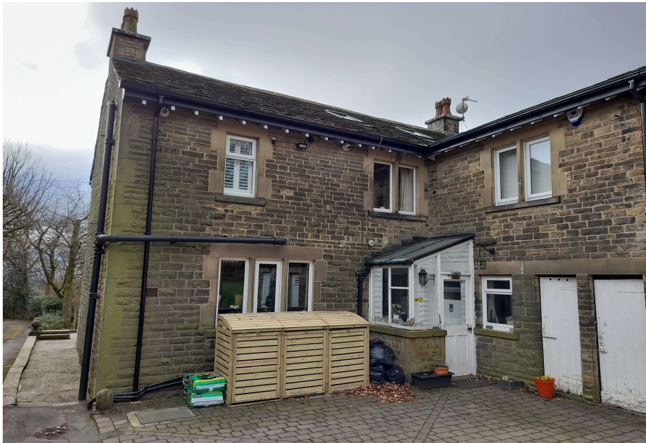
view of existing part northern elevation .
