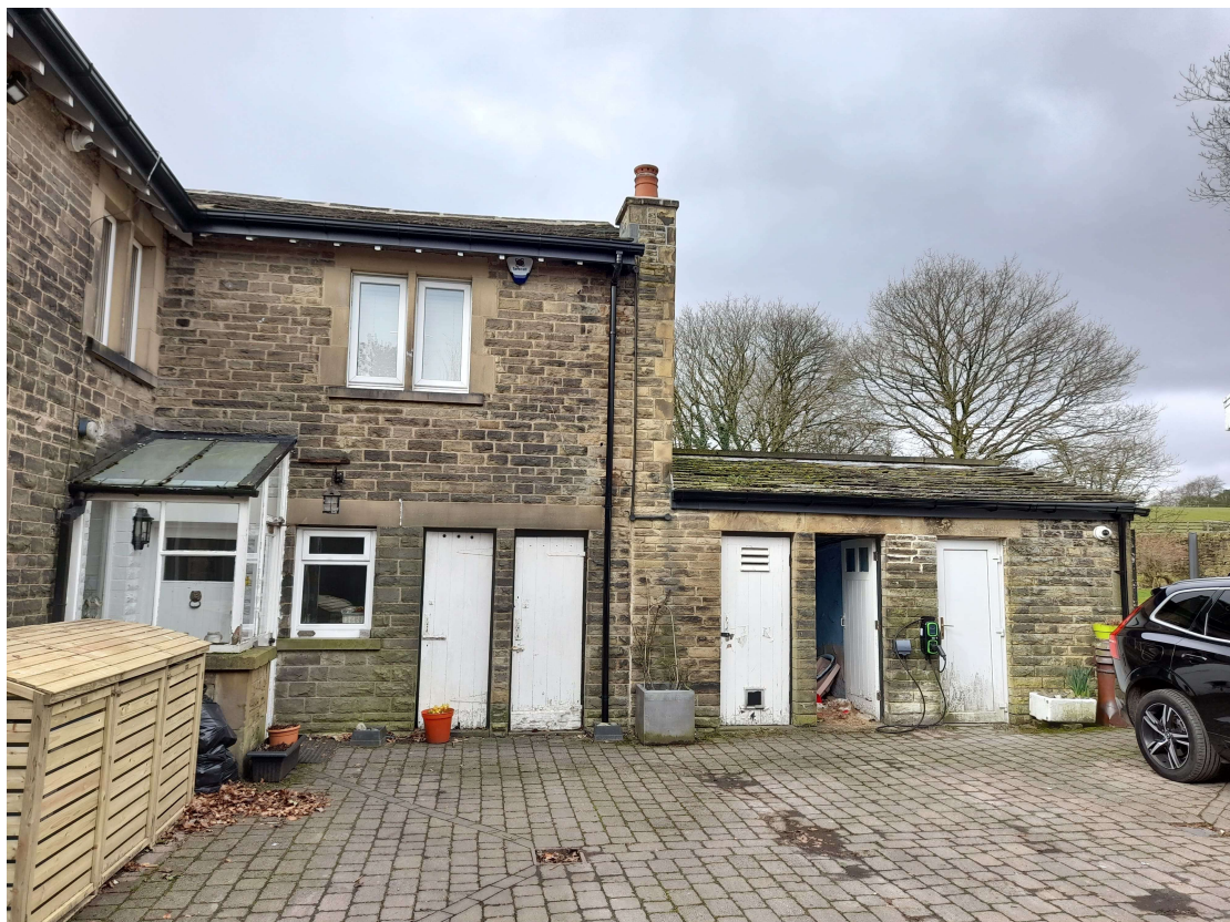
view of existing part western elevation .
