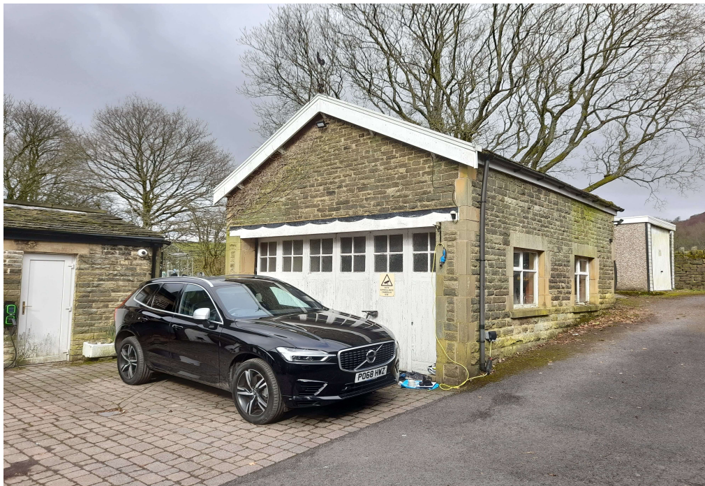
View of Garage to the north of extension site
