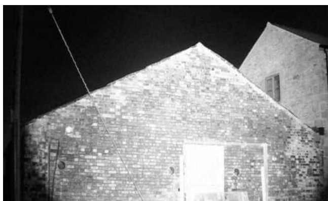
Northern Gable End
