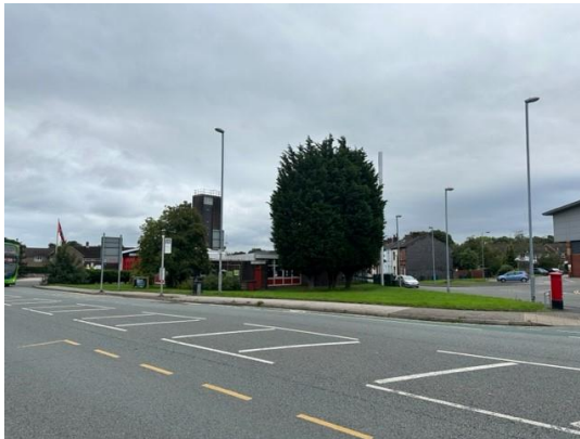
Figure 4: View of the site from Bury New Road
