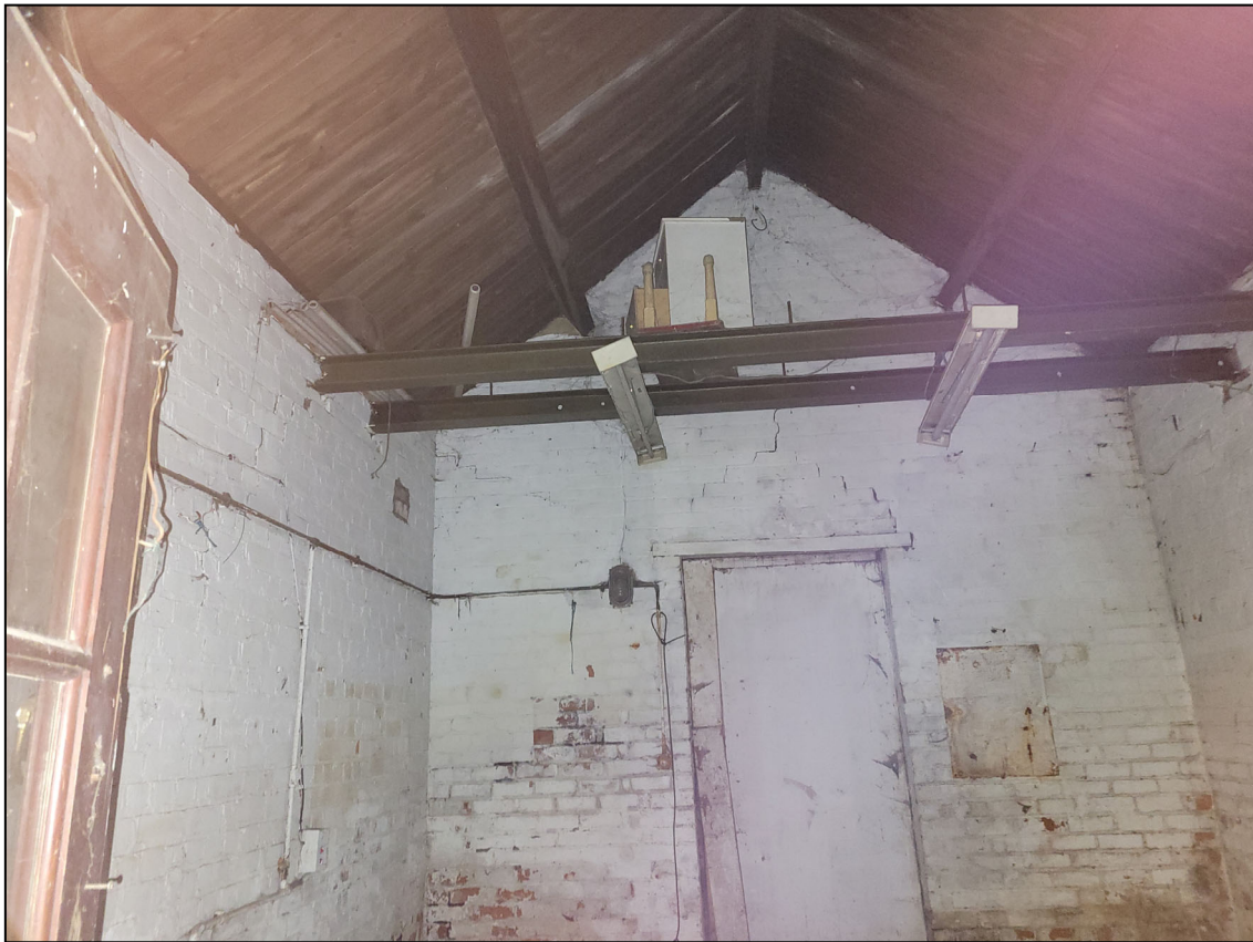
Photo 1 The building interior
