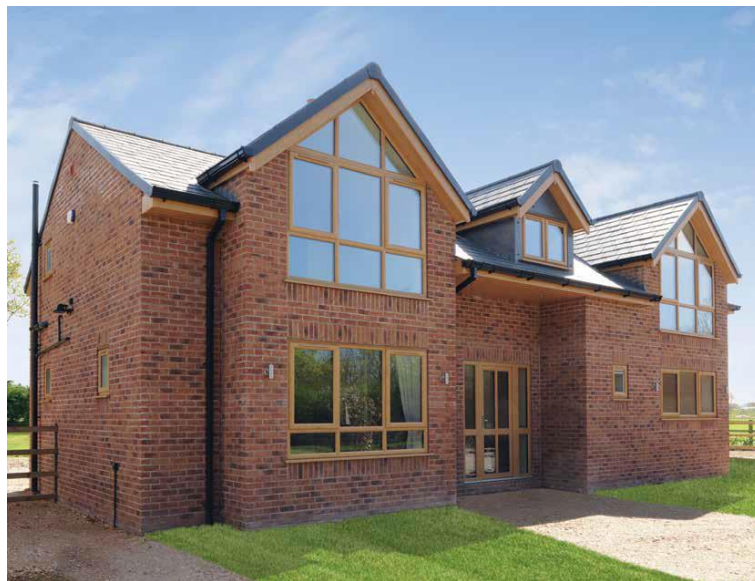
Image 4 – uPVC windows & doors
