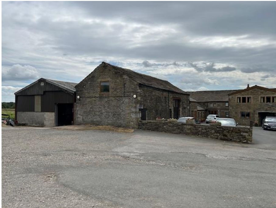
Image 2 – View to gable and front elevations of stone barn
