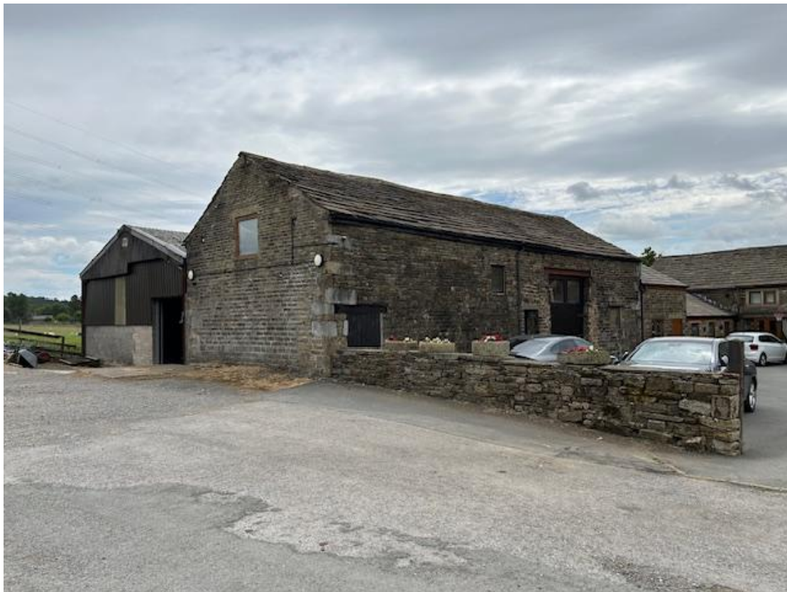
Image 1 – Existing stone barn and steel framed stables building
