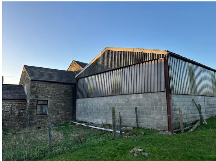
Image 4 – Rear of stone barn and steel framed building
