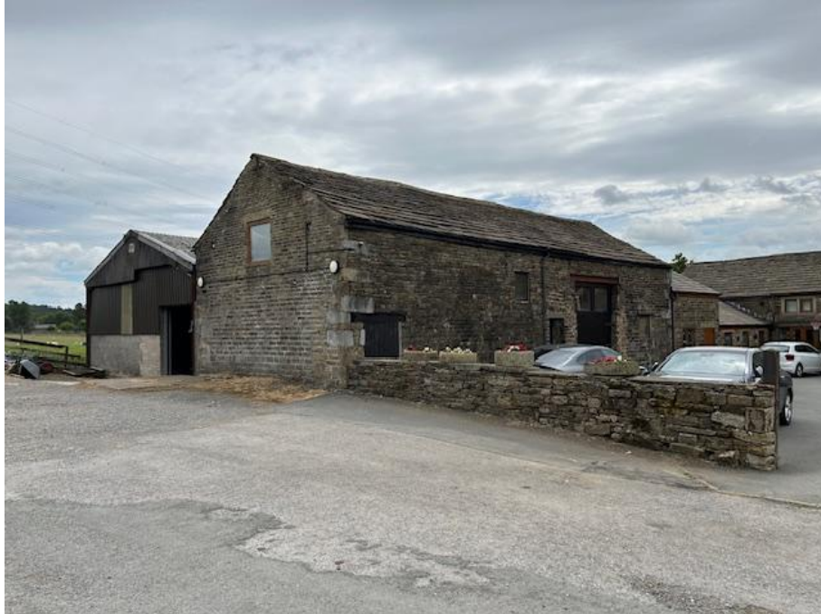
Image 2 - Existing stone barn and steel framed stables building
