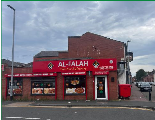
The northwest elevation of Structure A
