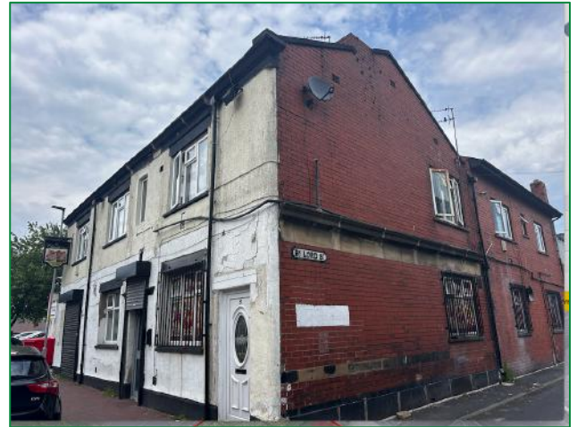
The southwest and southeast elevation of Structure B
