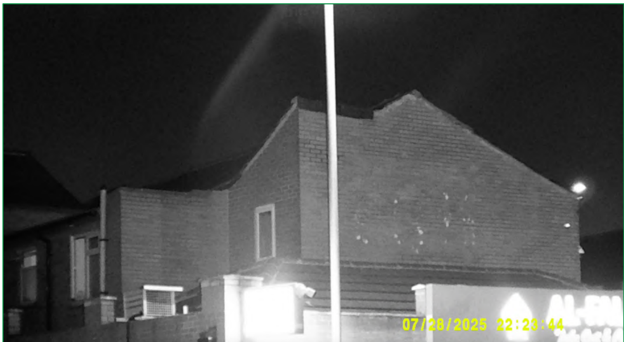
Showing the north elevation of the Structure B using the night vision aid.
