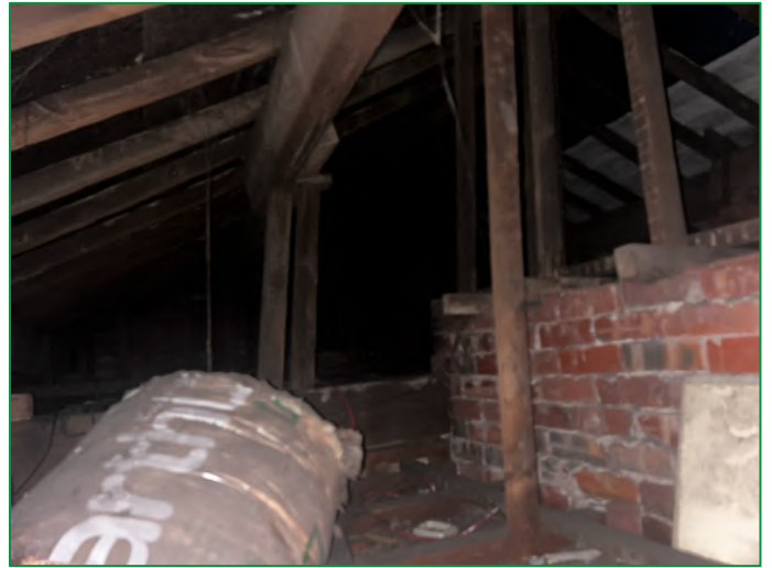
The loft void of Structure B
