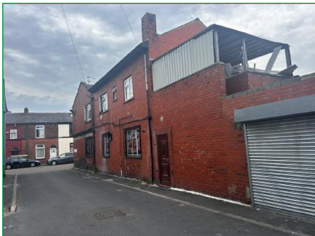
The southeast and northeast elevation of Structure C
