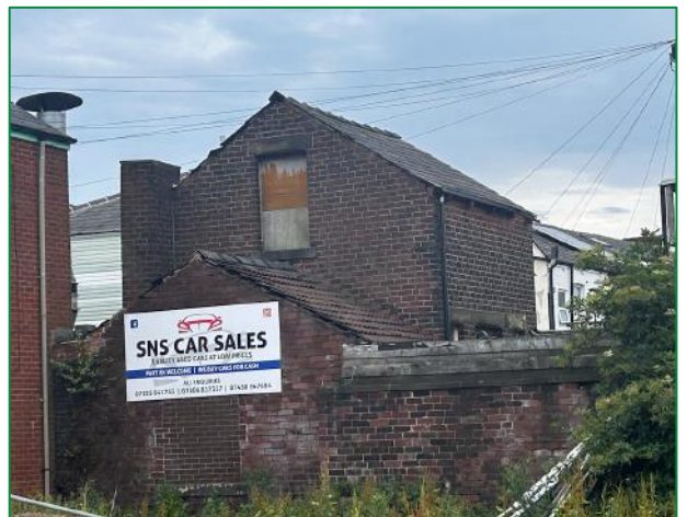
The northwest elevation of Structure D
