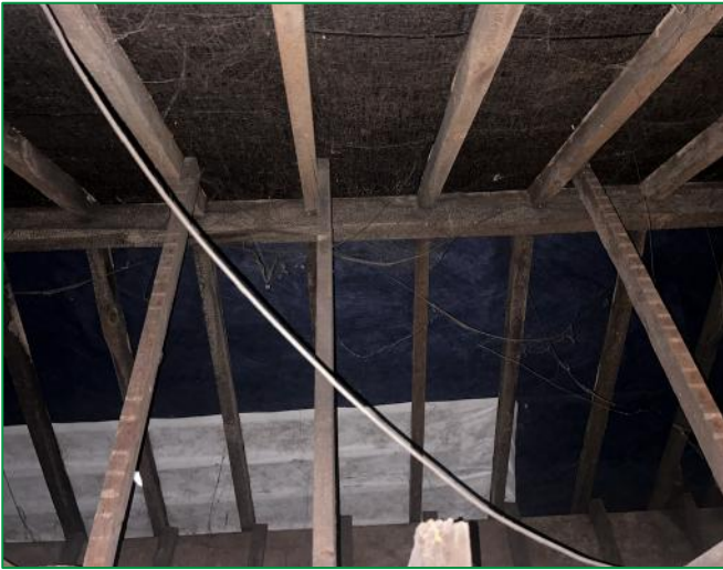
Showing exposed ridge beam in the loft of Structure B and dense cobwebs
