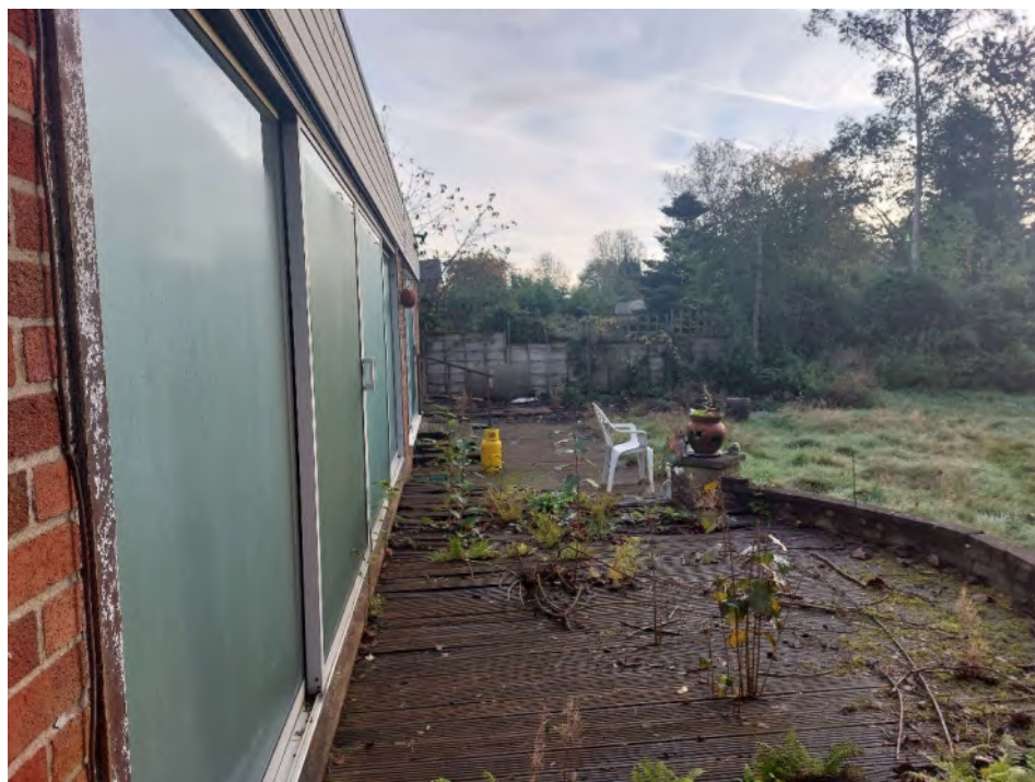
Photo 4 – Rear of existing property
