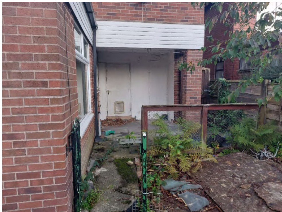
Photo 5 – rear access into existing property
