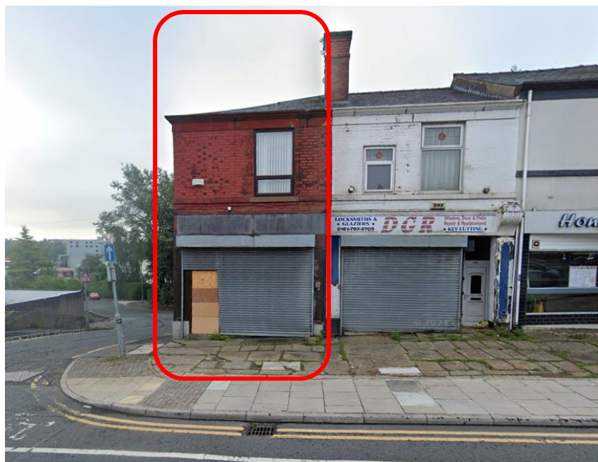
Figure 1 The application site
