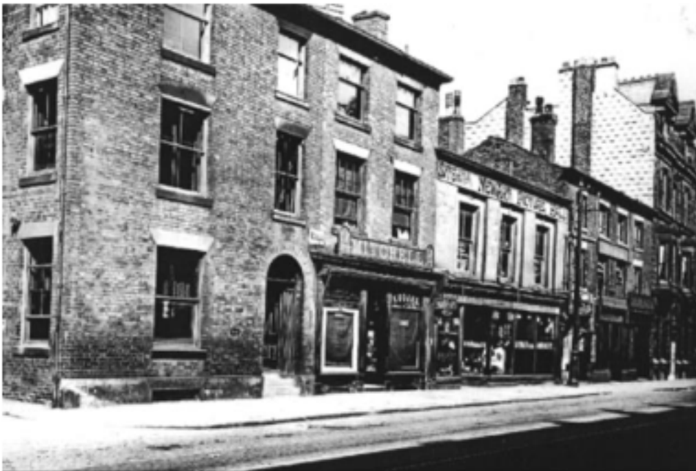
Image of application site building, 16-8 Bolton Street, 1895 | Bury Library archives
