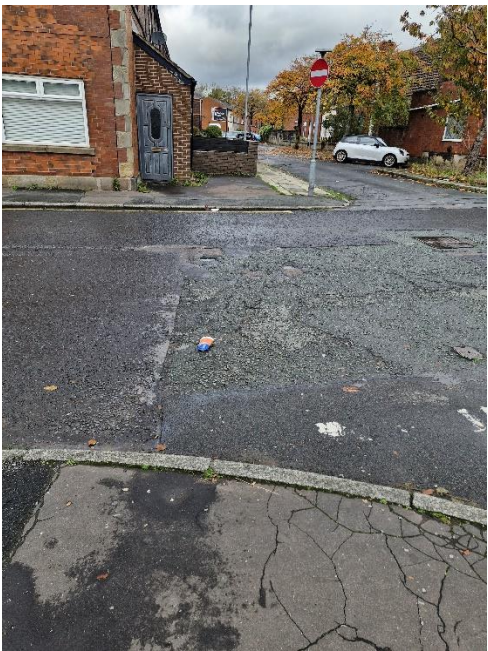
carriageway at Chesham St/Hilton St
