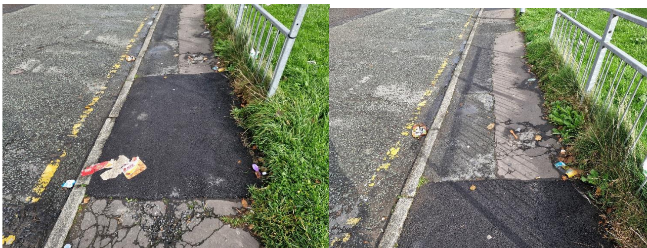
Chesham Rd footway looking east
