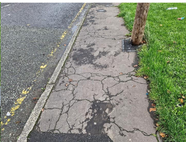
Footway near telegraph/BRSK(?) pole.
