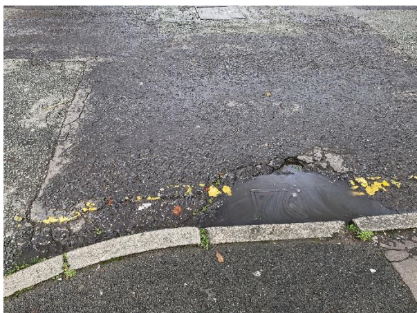
Junction back Walmersley Rd with Chesham Rd, badly deteriorated road markings, poor carriageway reinstatement and damage to carriageway.
