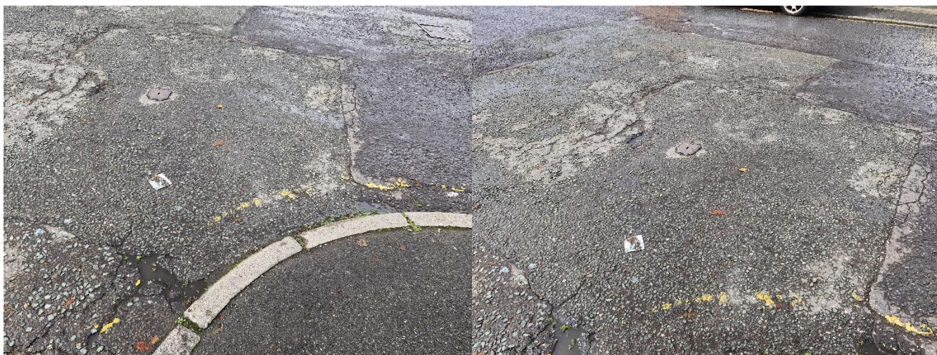
Junction back Walmersley Rd with Chesham Rd, badly deteriorated road markings, poor carriageway reinstatement and damage to carriageway.
