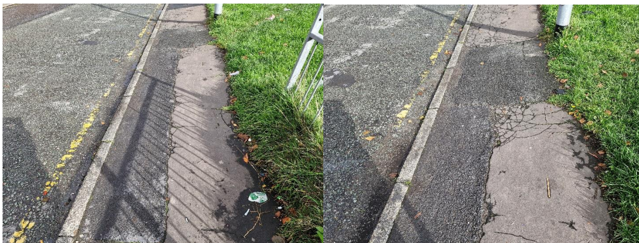
Looking east, reinstatement following LC installation.
