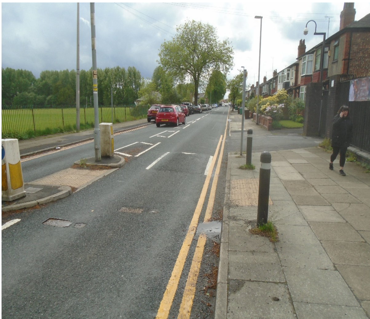
PHOTO 5 : Looking down Park Lane from the school entrance showing parking to the left-hand side with a lot of cars parking half onto the public footpath.
