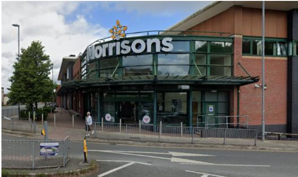
Entrance to Morrisons at the corner of Bury New Road/Stanley Road
