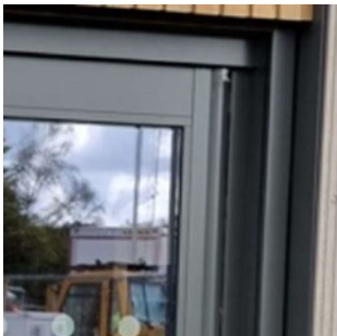
Glazing and Doors Umbra grey aluminium frames
