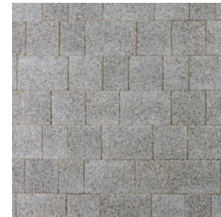
New Paving to Building Grey Block Paving
