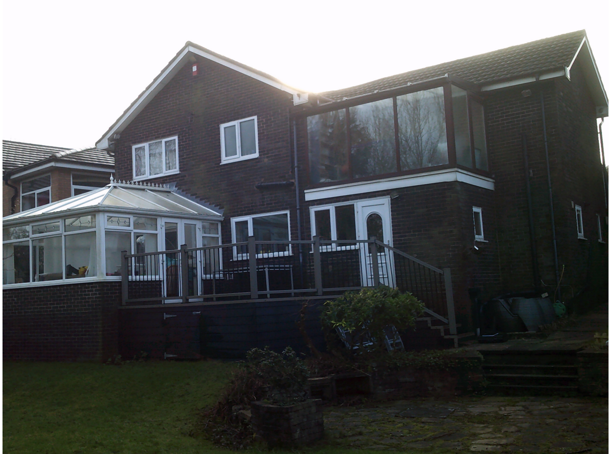
View to rear of property
