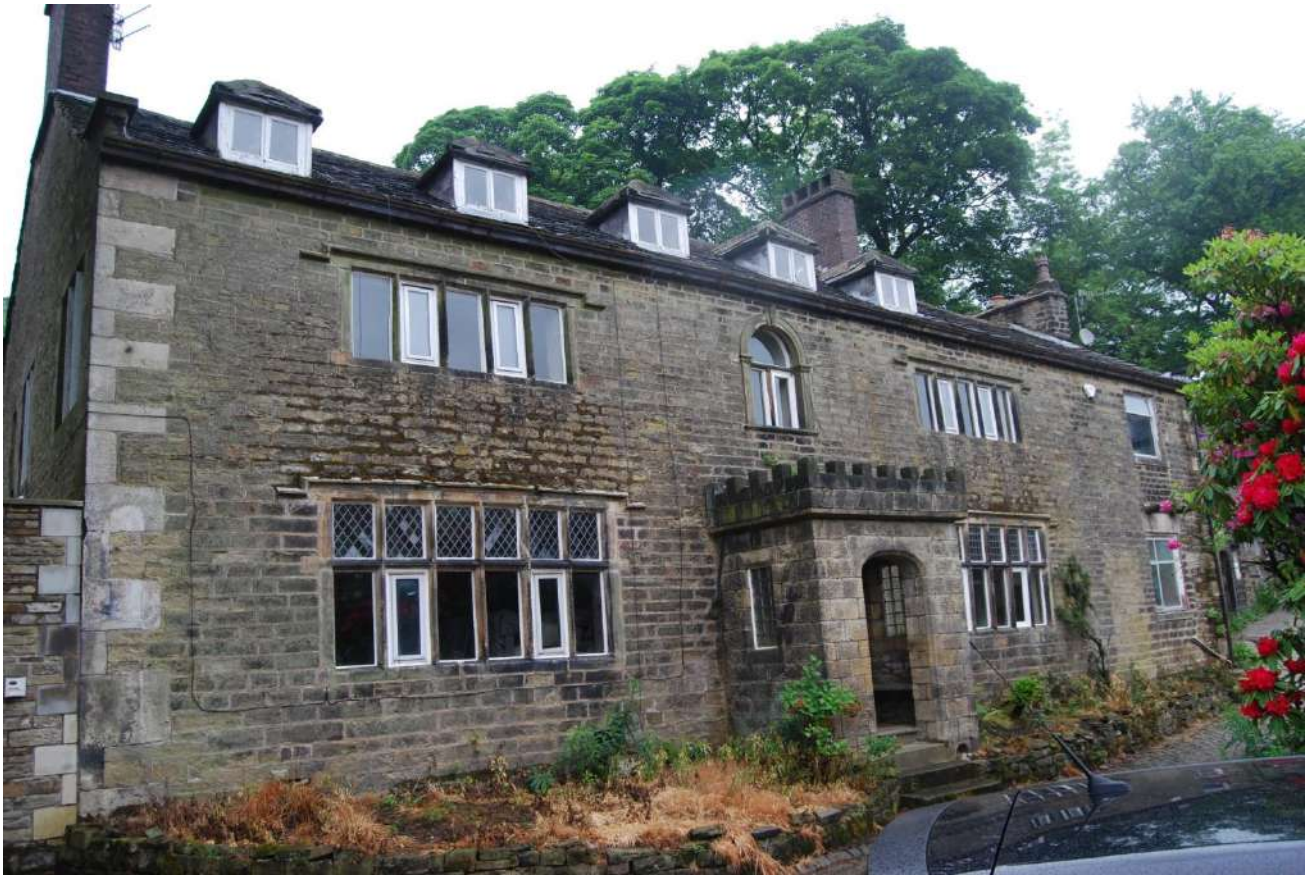
Figure 2. View of the property from the Moor Road. Illustrates the general coursed stone construction, later porch addition, ashlar features and dormers.
