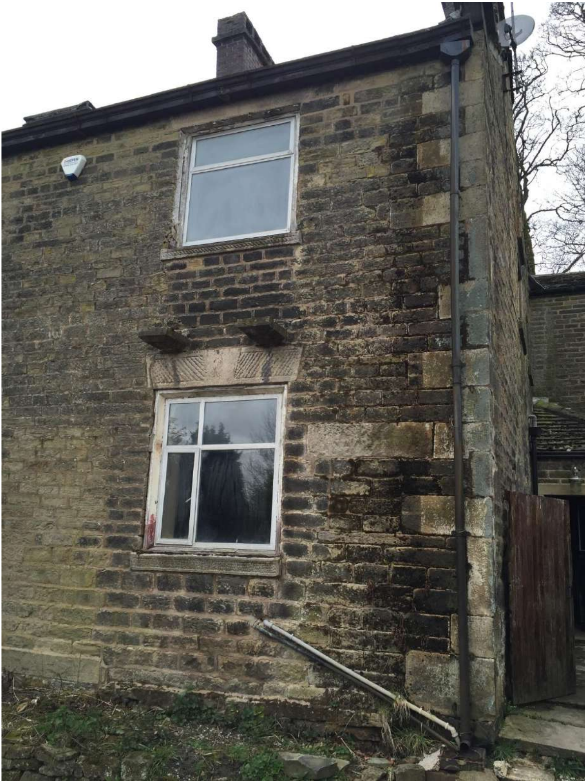
Figure 3. The Manor House was extended to the north in 1820 with alternative stone detailing. The stone corbels of an original Juliet balcony remain.
