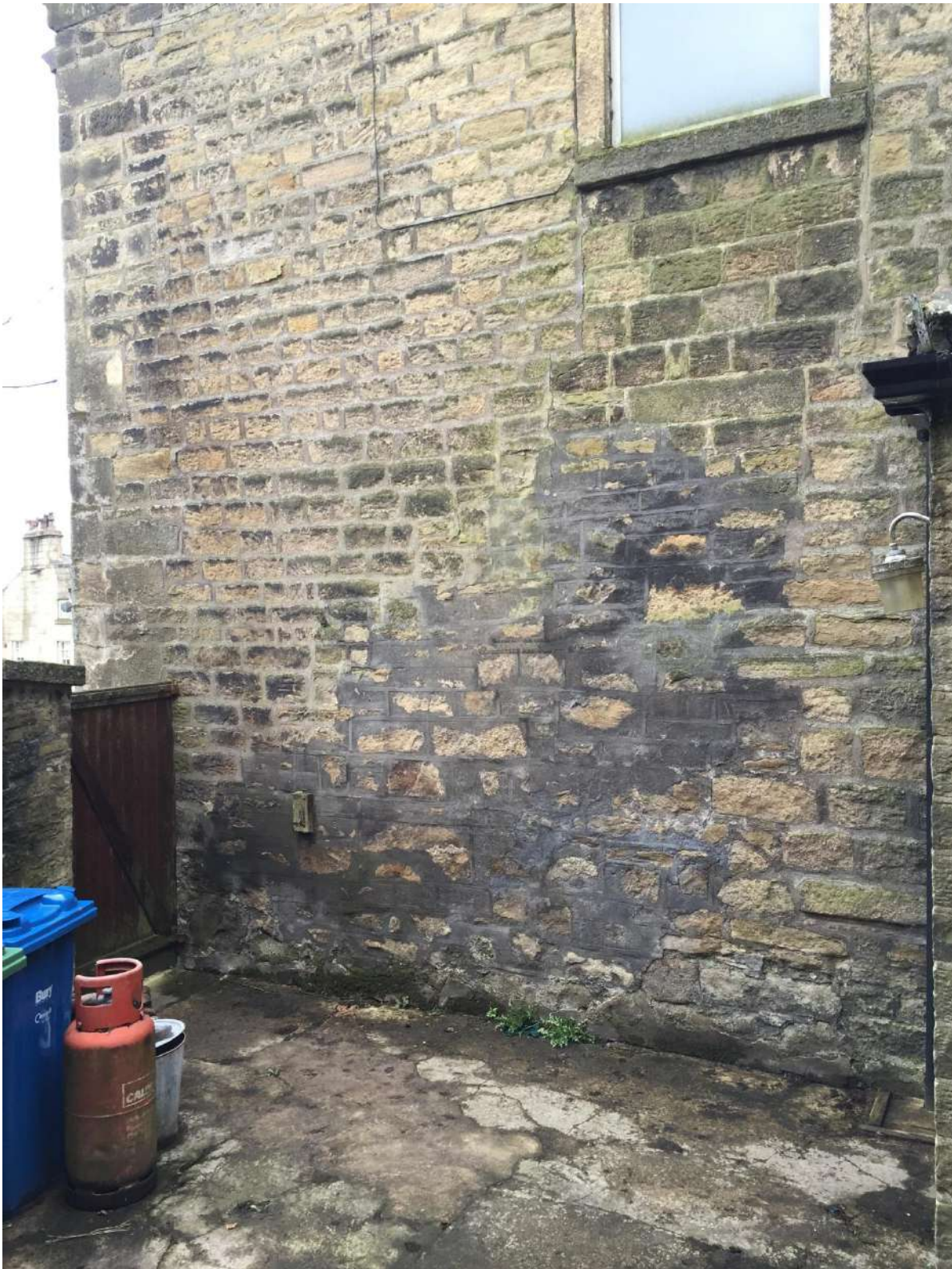
Figure 11. North gable wall with a combination of coursed and random stone indicating previous modifications.
