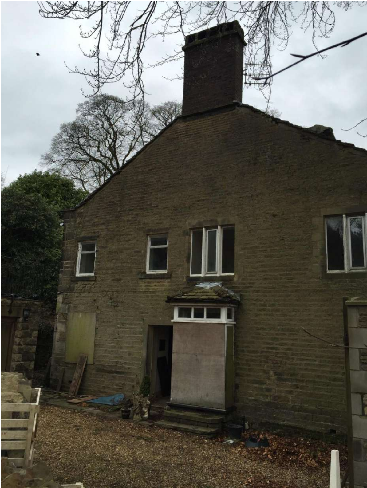
Figure 4. South gable wall. Illustrates stone coursed construction, bay window at ground floor level. Also note imposing brick chimney.
