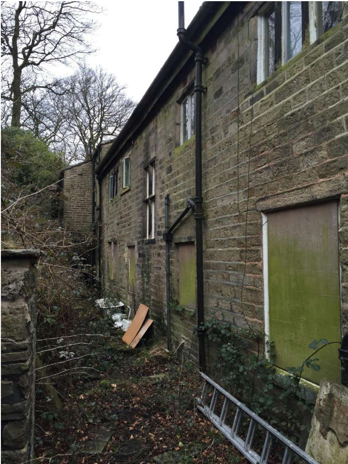
Figure 5. West elevation (to the rear). Illustrates stone construction with stone lintels and cills. Note feature stair window with central stone cross and four light window.
