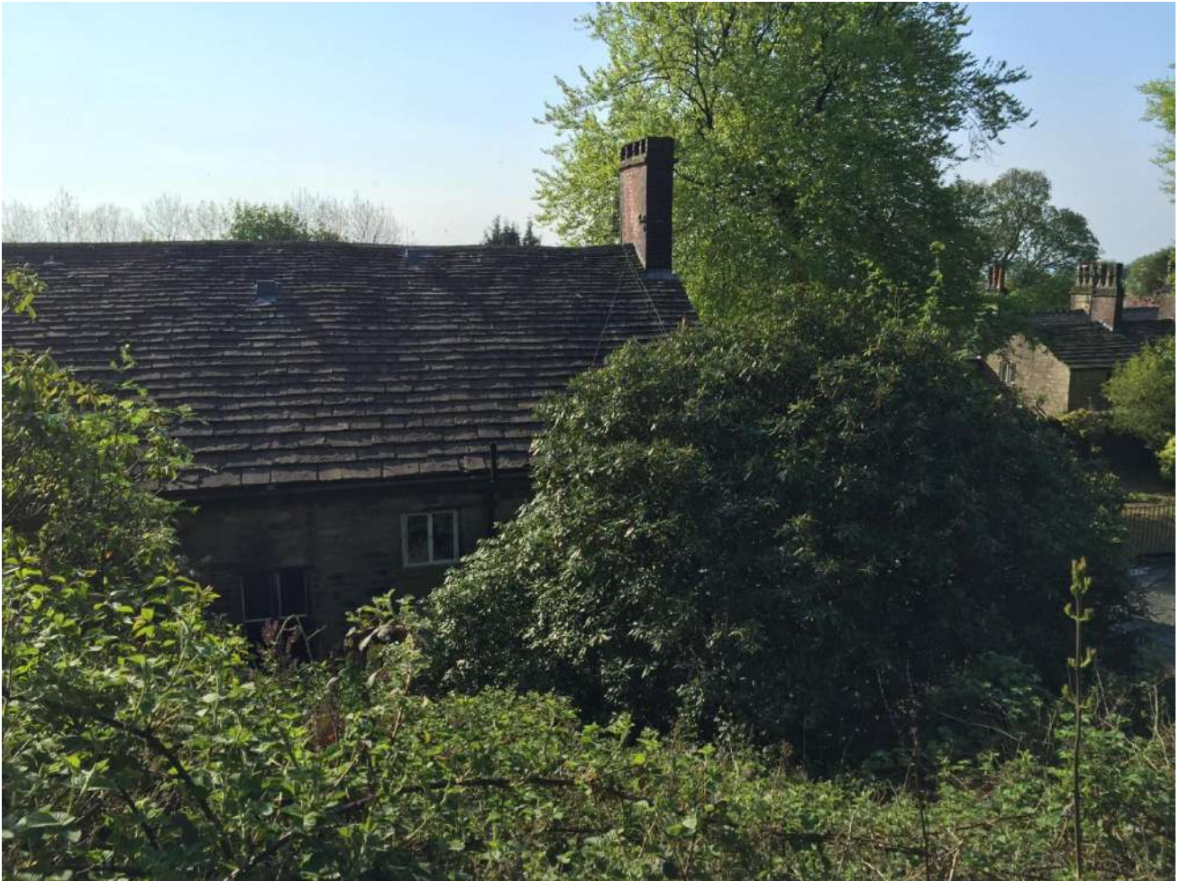
Figure 9. View of the rear elevation and roof looking east from Holcombe Moor.
