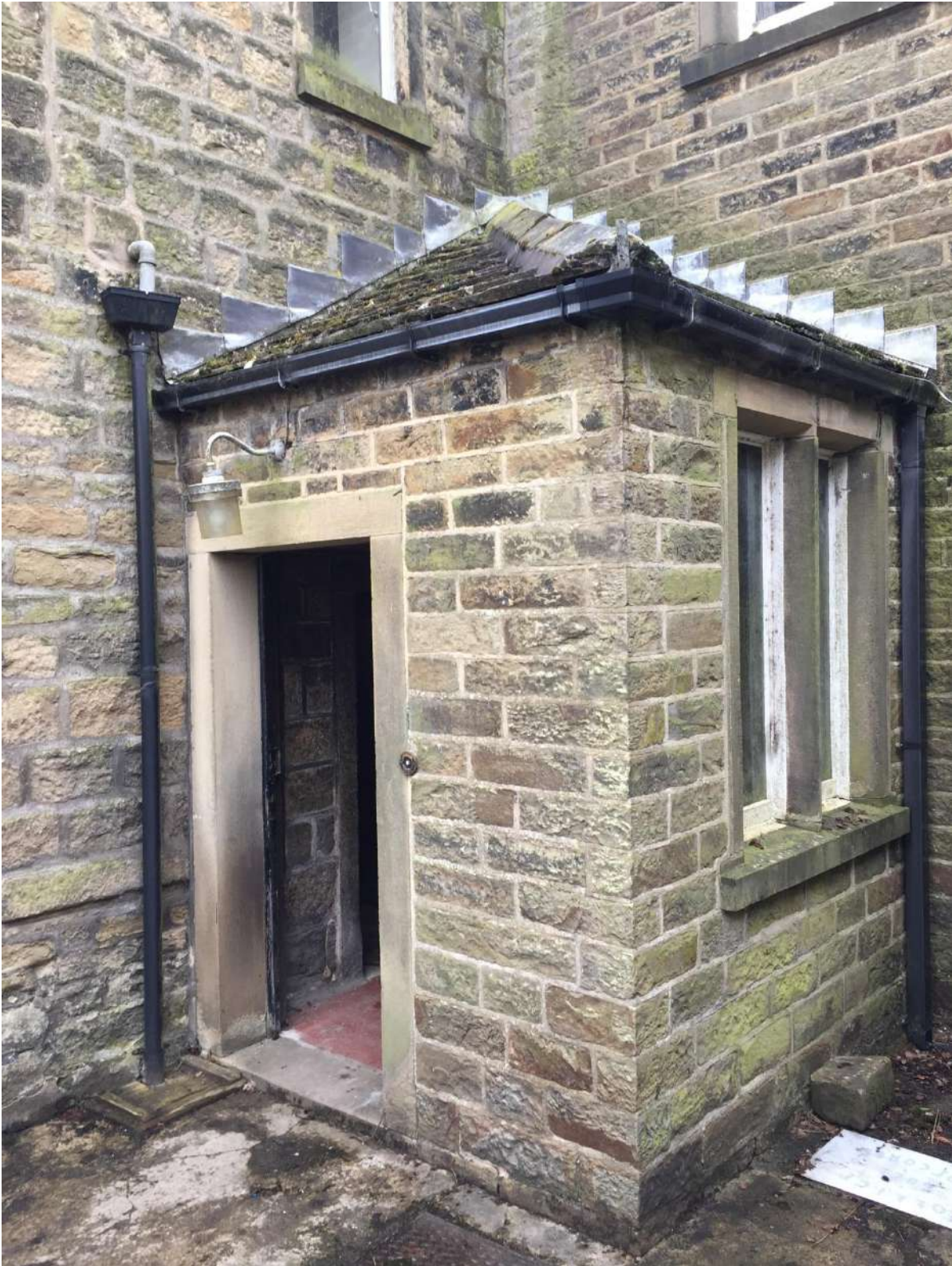
Figure 12. Later addition single storey stone porch pre 1930.
