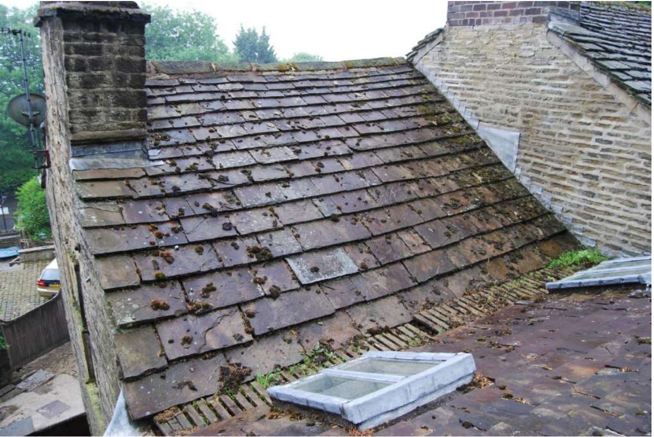
Figure 14. Roofscape looking east over the later 1820 addition.
