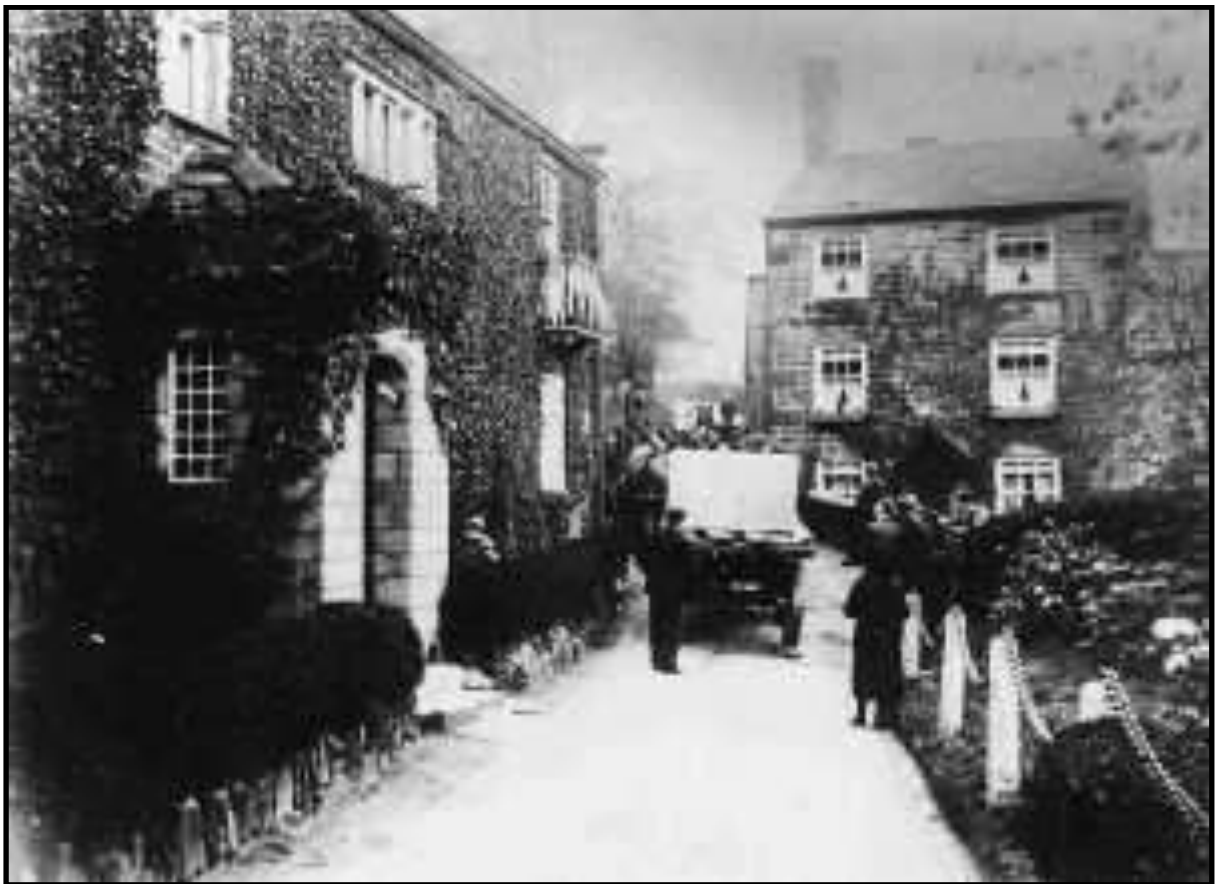
Figure 51. Frontage showing original Juliet balcony supported on stone corbels dated 1902 (Photo from Ramsbottom Heritage Society Photograph Achieve)
