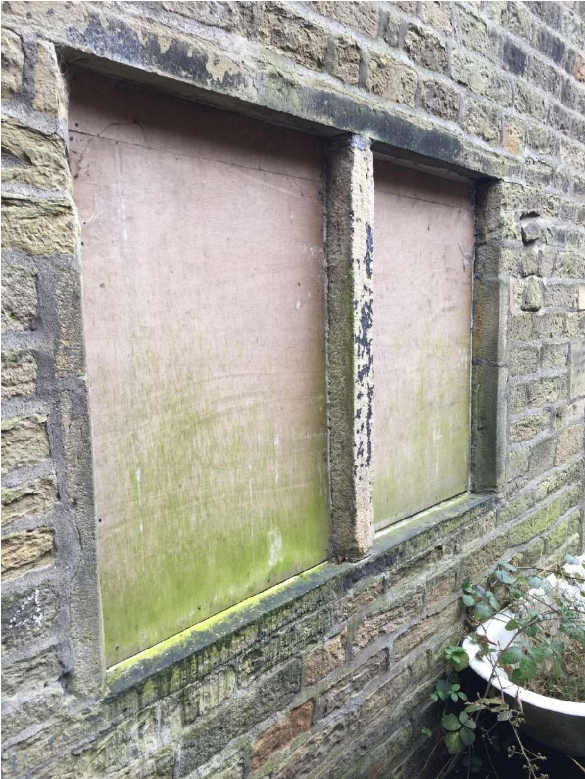
Figure 8. View of stone window whose head height has been raised leaving the original stone jambs in place.
