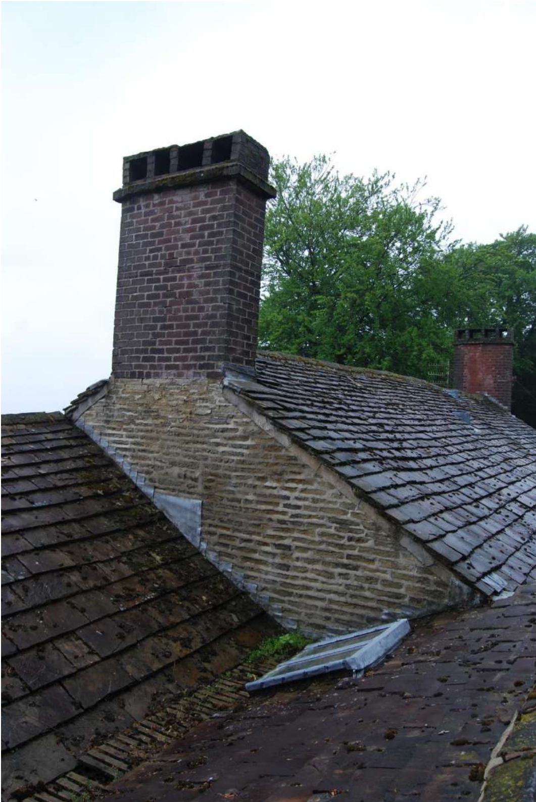
Figure 13. Roofscape looking south. Note original gable abutment of the original manor house and imposing brick chimneys. We believe the large lead flashing covers a former staircase opening which was used for staff / servants.
