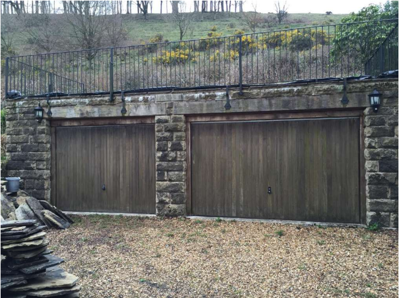
Figure 16. Single storey garage with roof terrace. Post 1960.
