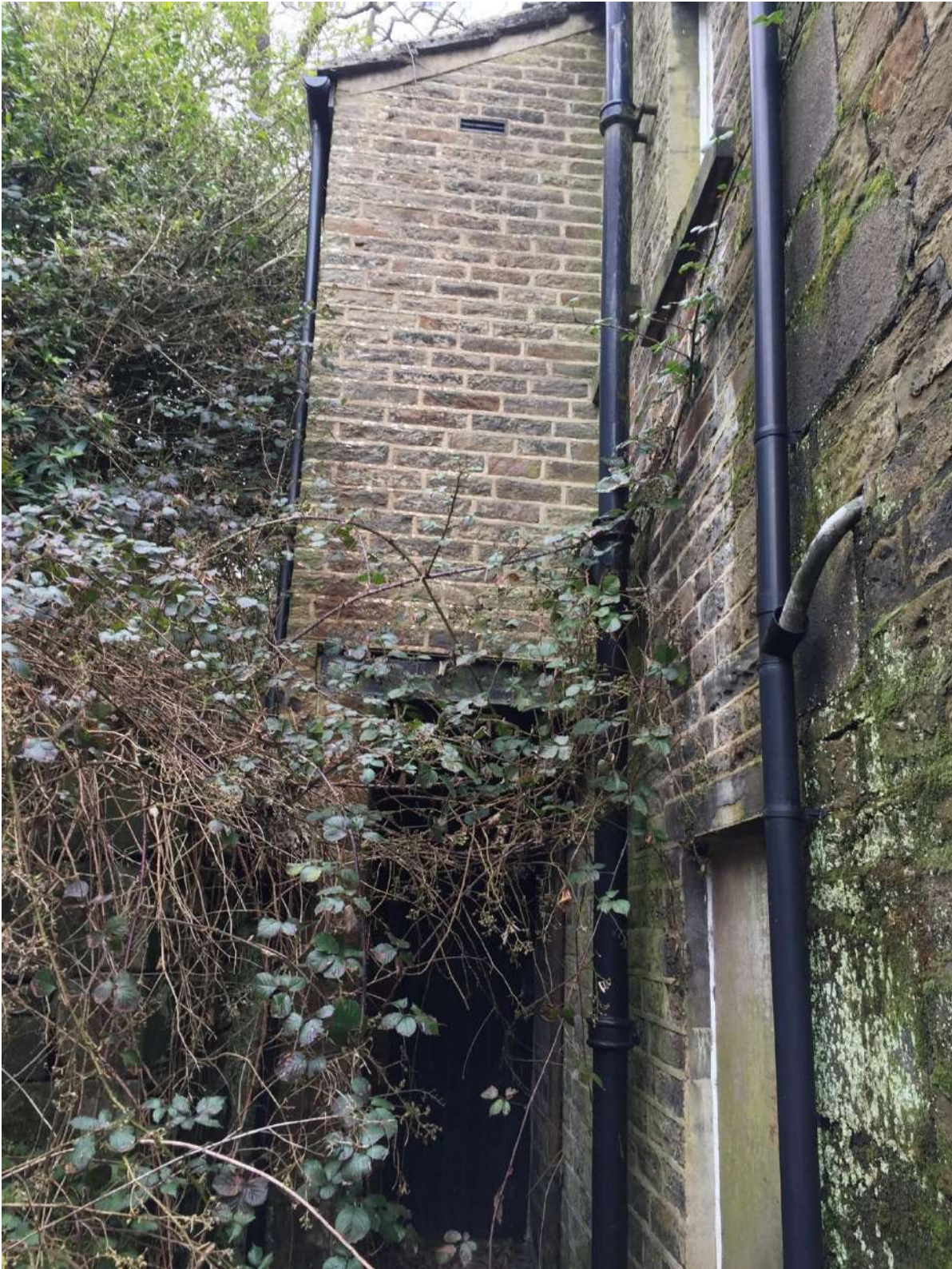
Figure 7. Note how the first floor extends over a covered area to the rear. Product of a later extension.
