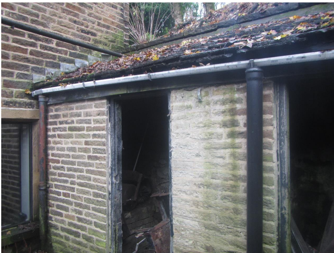
Photograph 16 – View of lead flashing on the eastern aspect of Building 4.
