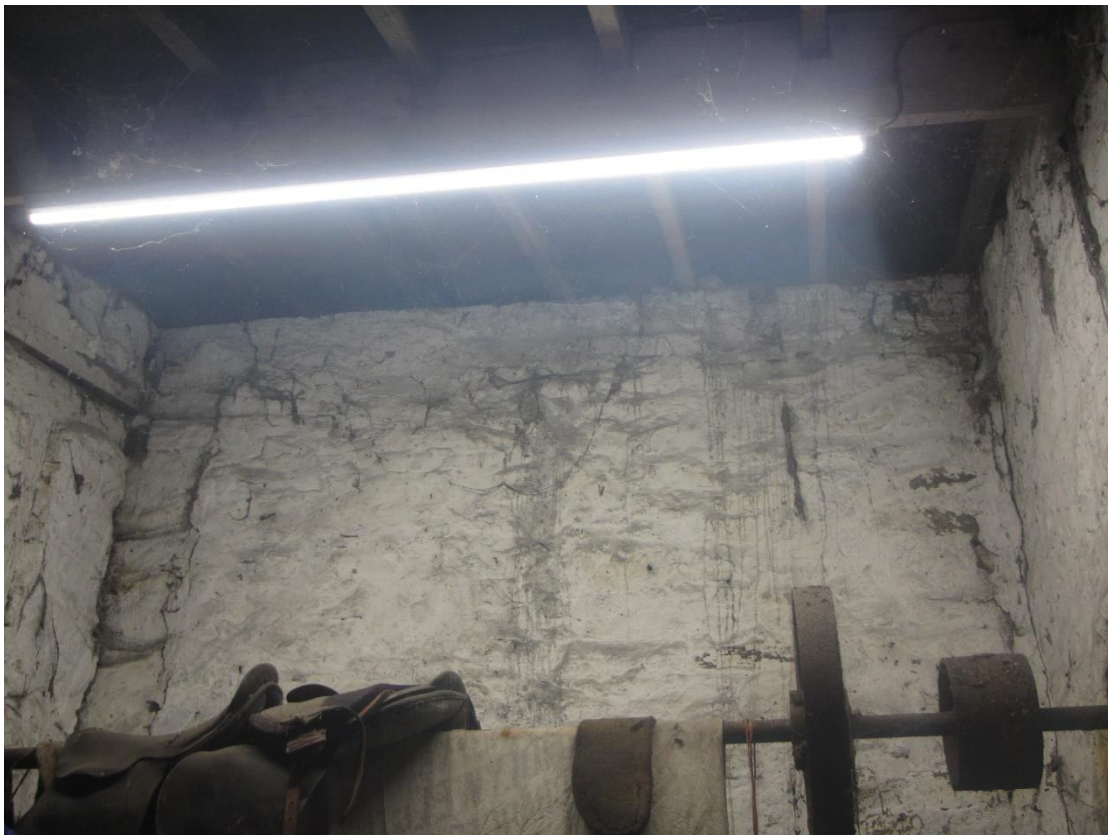
Photograph 20 – Internal view of Section A within Building 2.
