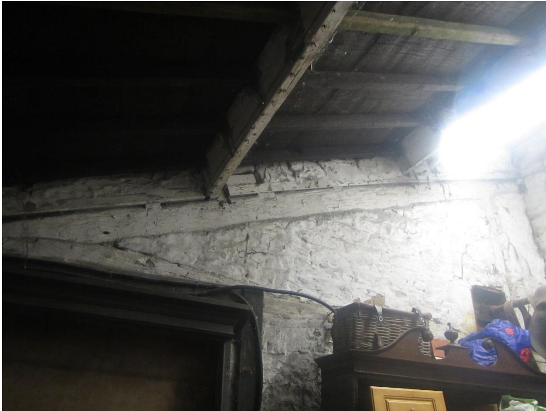
Photograph 21– Internal view of Section A within Building 2.
