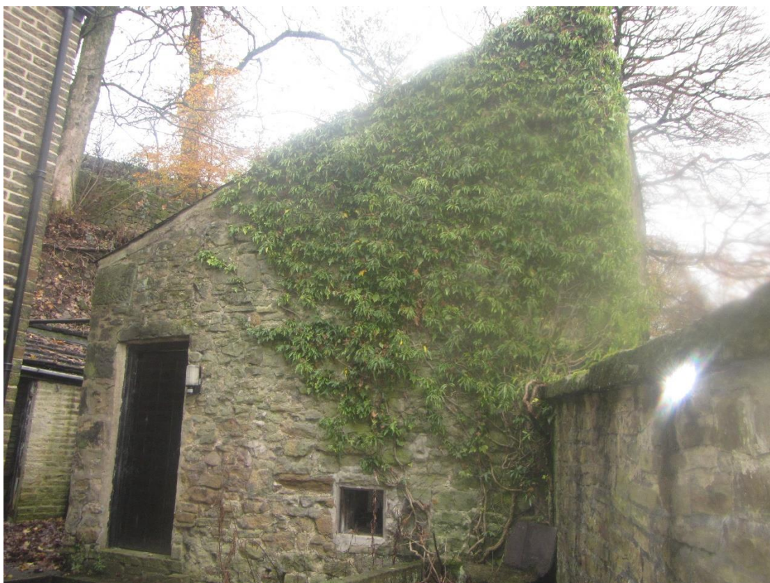
Photograph 11 – South-western aspect of Building 2.
