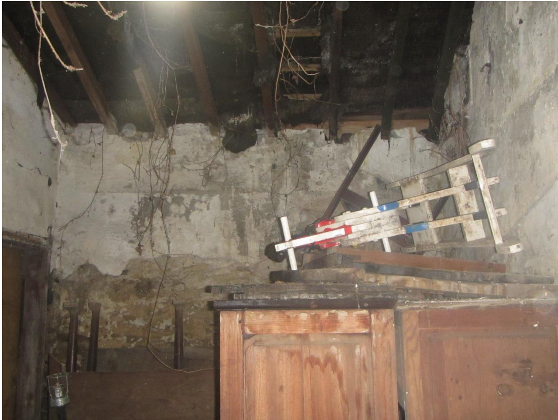
Photograph 25 – Internal view of Section B within Building 2.
