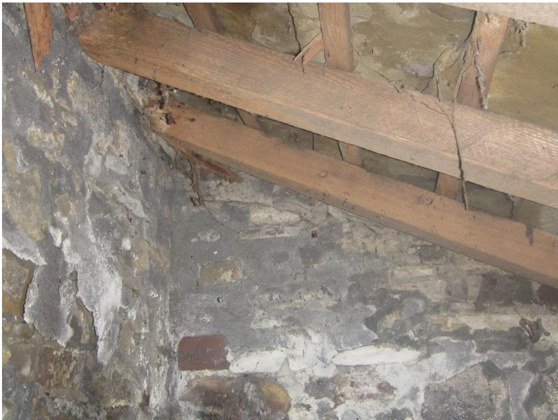
Photograph 18 – Internal view of Building 1.
