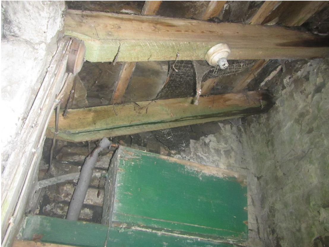
Photograph 30 – Internal view of Building 4.
