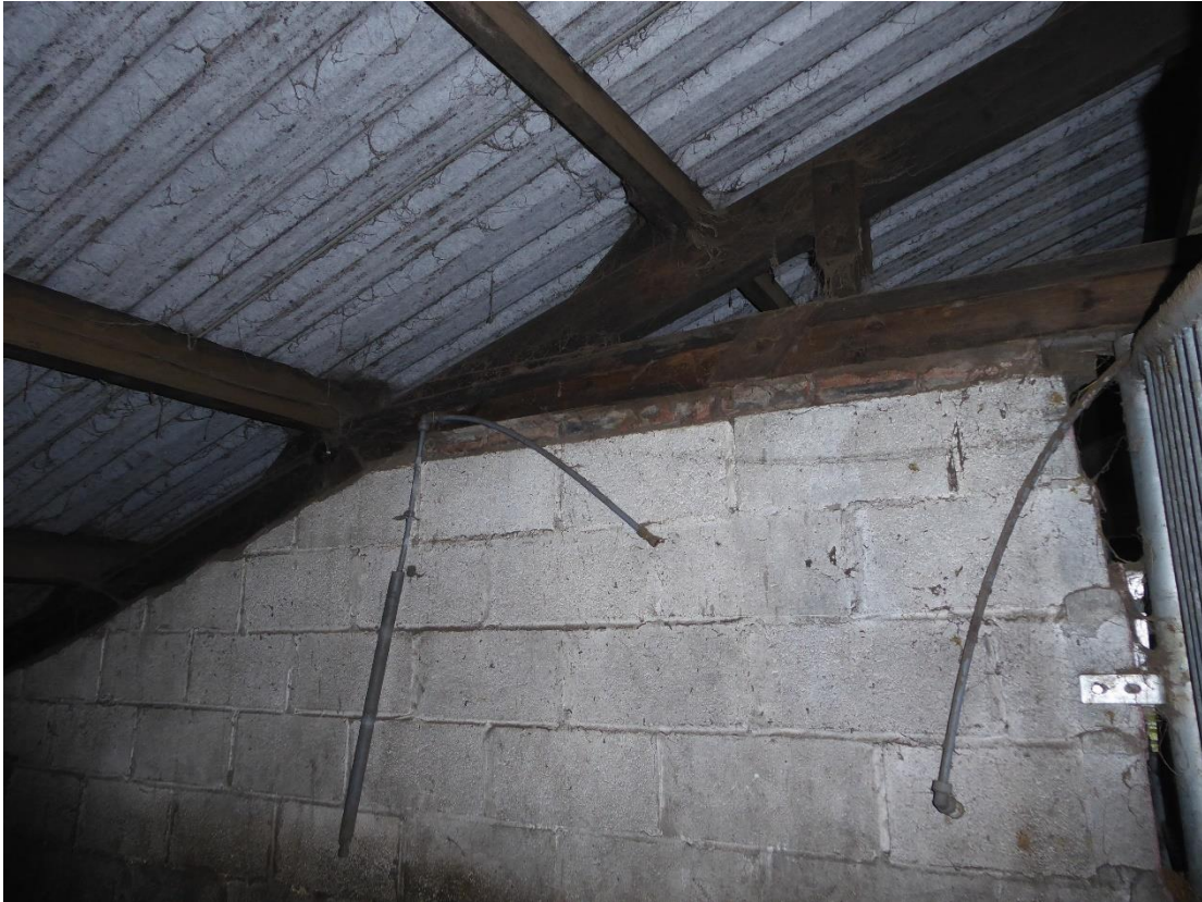
Photograph 4 – Partial view of the internal supporting masonry walls.
