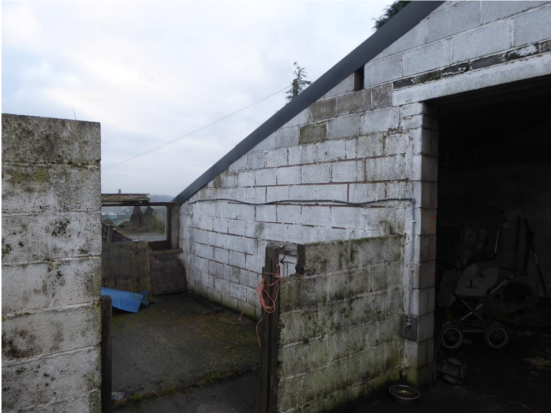
Photograph 2 – Partial view of the southern elevation.
