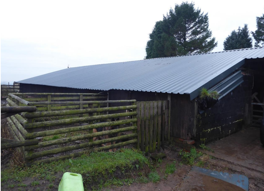
Photograph 1 - General external view of the eastern elevation.
