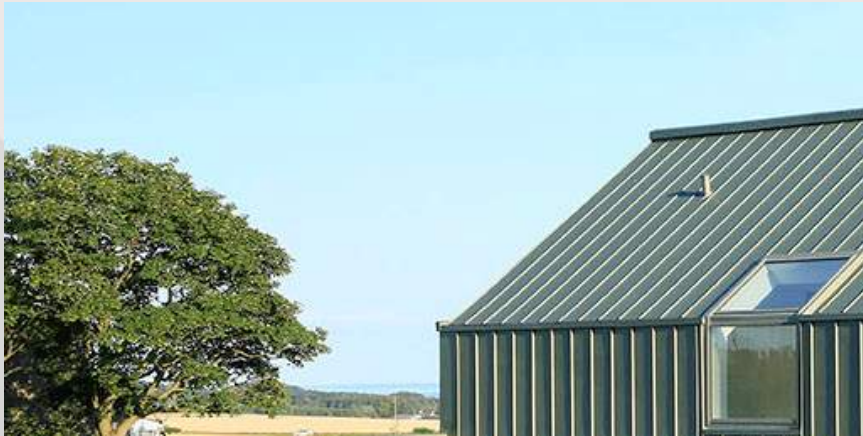
Image 7. Green Zinc Cladding used in Greenbelt.
