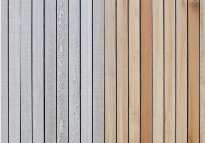
Image 4. Weathering natural timber vertical cladding.
