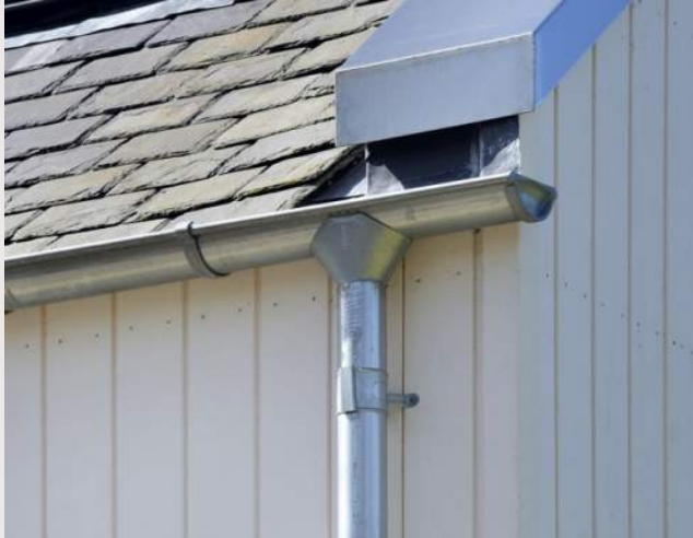
Image 8. Zinc rainwater goods (will be Lichen Green).
