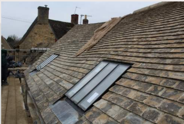
Image 9. Conservation, all metal skylights.
