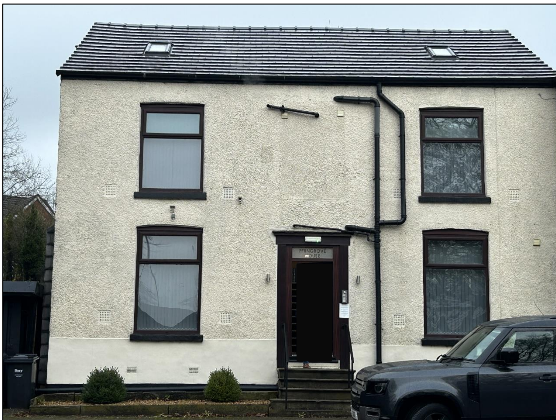
Plate 1 – The southern elevation of B1 on site
