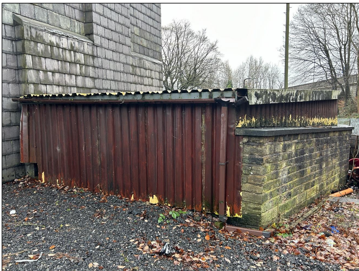
Plate 10 – Northern and western aspects of B2
