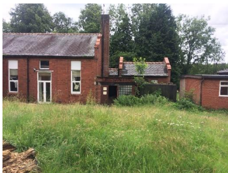
Photograph 5 (P5) Site from centre looking southwards. Fuel tank can be seen in the middle of picture. Ground in the area was tarmac.
