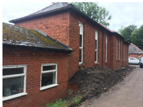
Photograph 4 (P4) Building (The Coach House) in the centre which is set lower than north of site. Tarmac is in good condition.
