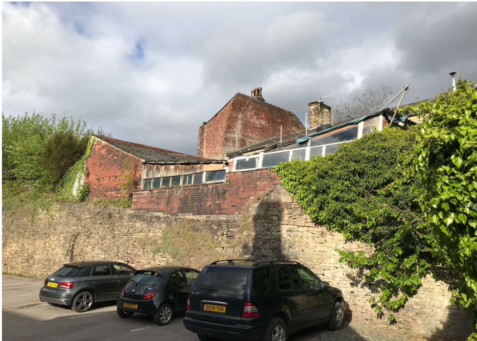
View of rear elevation prior to demolition works.
