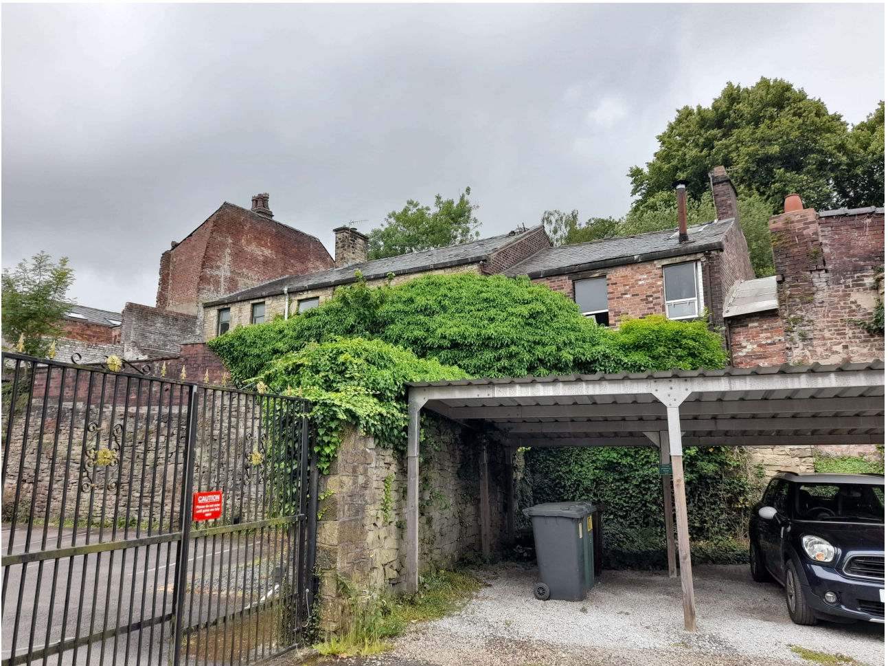
View of eastern elevation from the only public accessible view point
