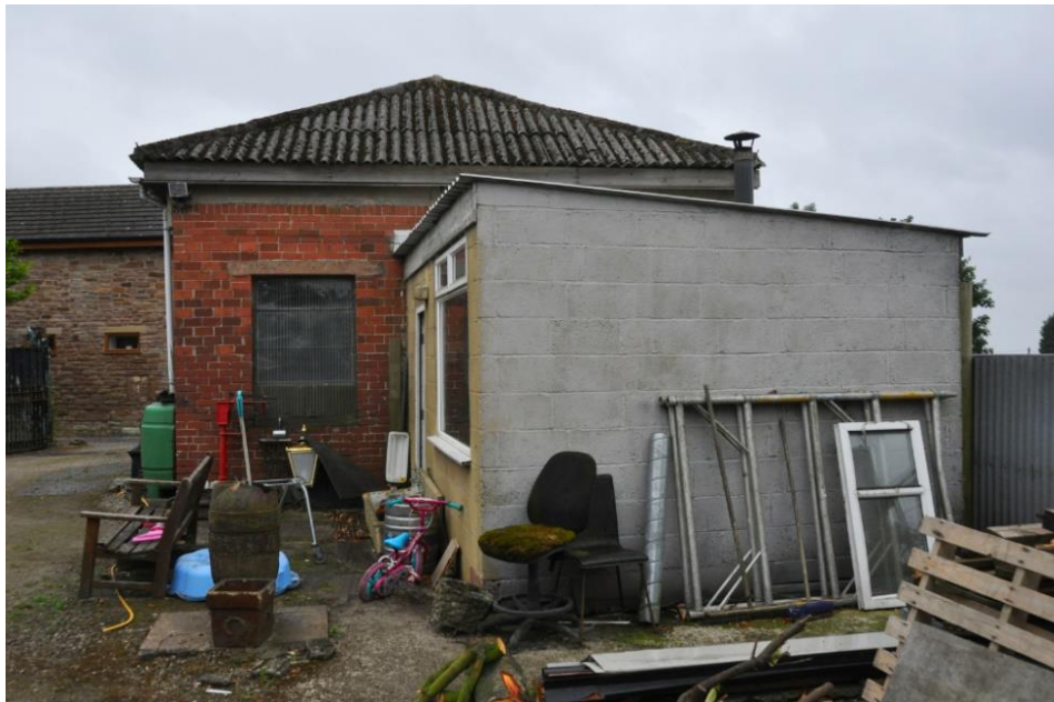
Image showing north elevation with main workshop in the background and adjoining flat roof extension in foreground
