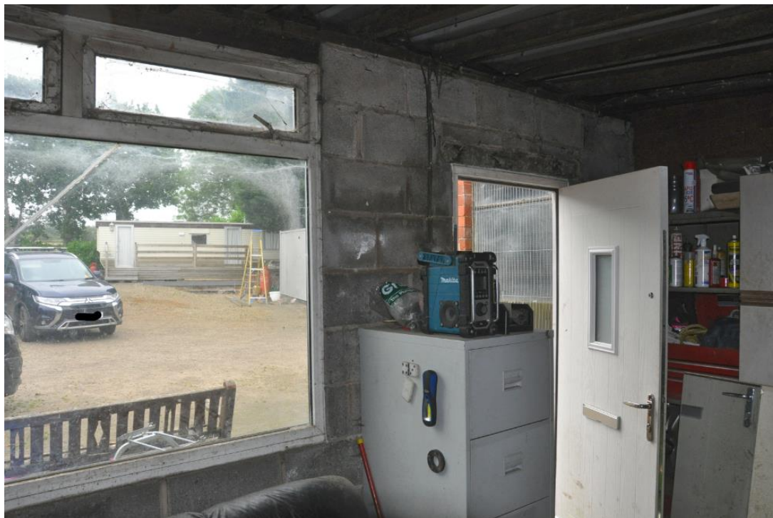
Image of showing interior of flat roof extension
