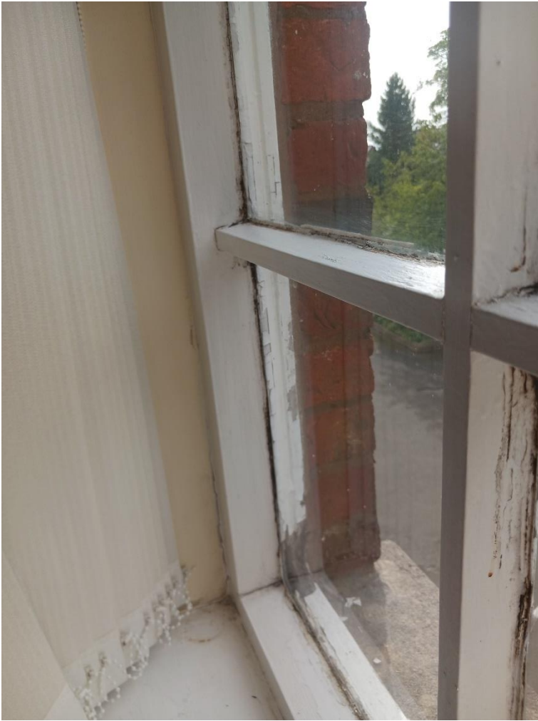
Figure 14: Detail of Central Window
