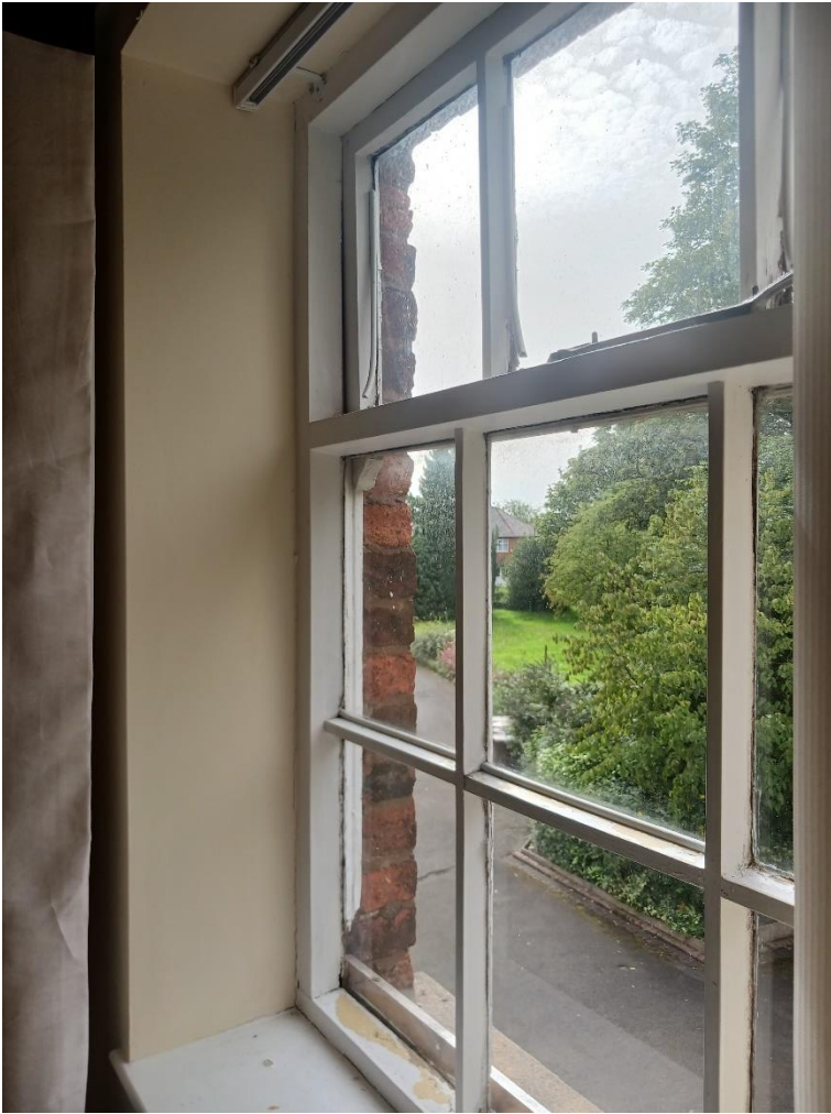
Figure 5: Detail of RHS window
