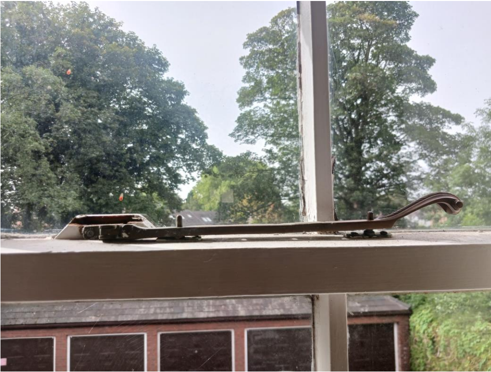
Figure 15: Detail of Central Window
