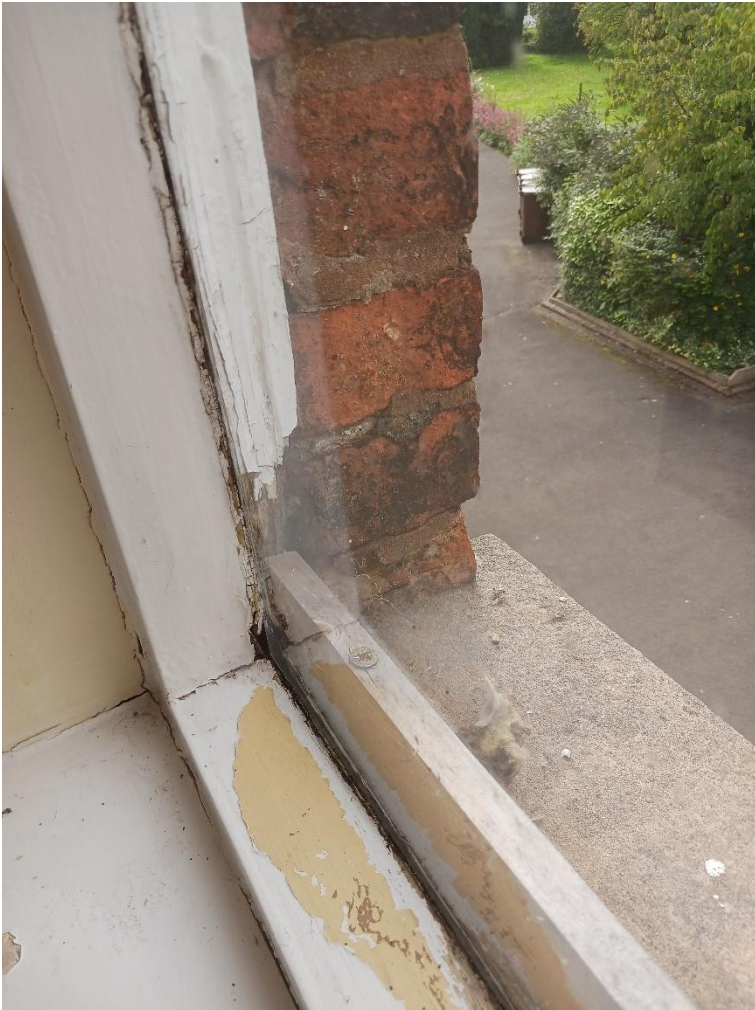
Figure 7: Detail of RHS window
