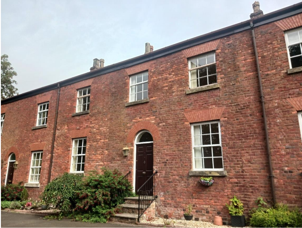
Figure 1: Frontage of 3 The Stables
