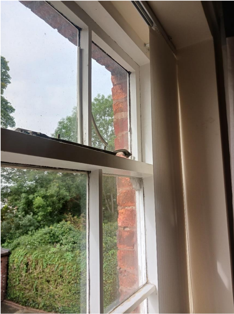
Figure 6: Detail of RHS Window
