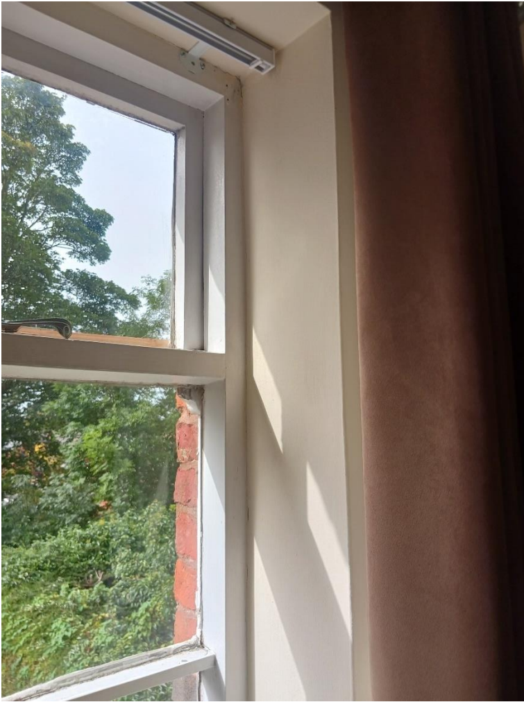
Figure 11: Detail of LHS Window
