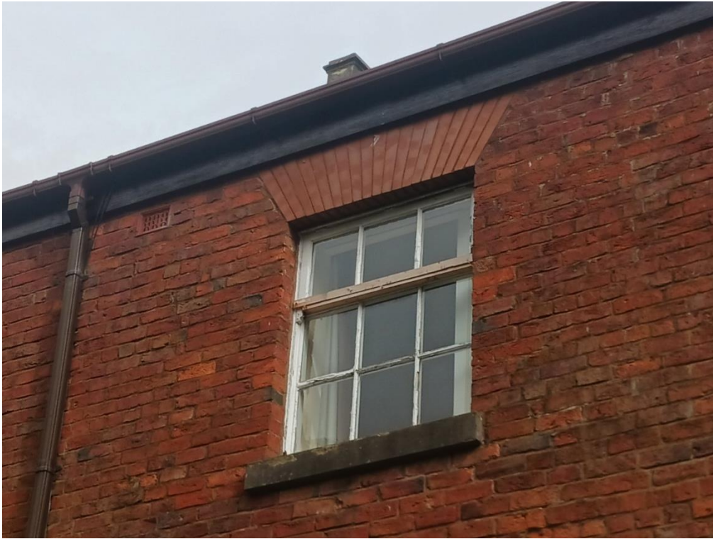
Figure 3: Detail of LHS window
