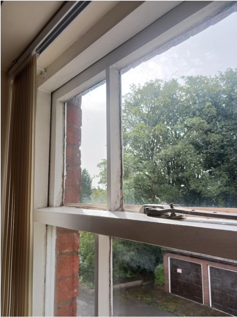
Figure 10: Detail of LHS Window
