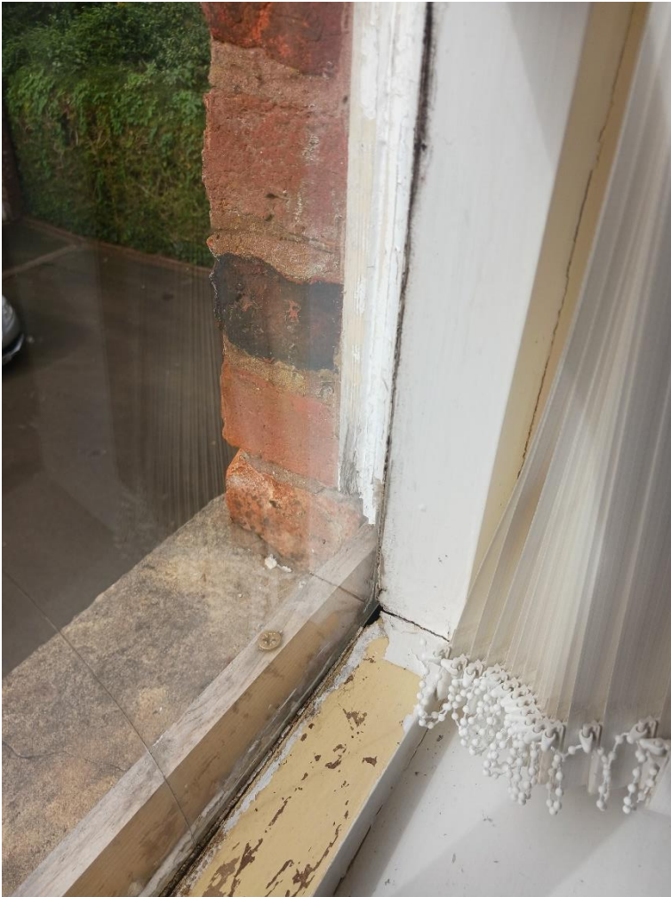
Figure 8: Detail of RHS window
