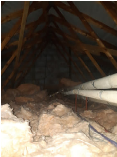
Photograph 9: Loft void in the Southern wing of building 1.
