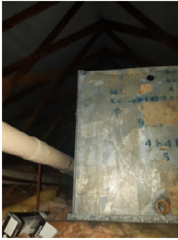
Photograph 7: Loft void in the Southern wing of building 1.
