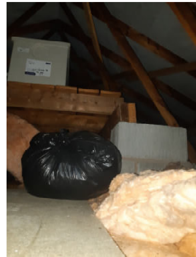
Photograph 10: Loft void in the Western wing of building 1.
