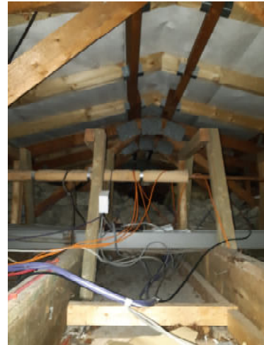
Photograph 6: Loft void in the Eastern wing of building 1.
