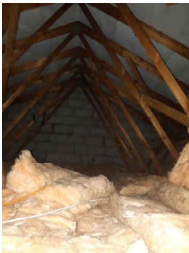
Photograph 11: Loft void in the Western wing of building 1.
