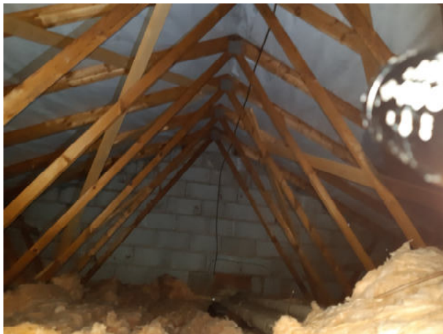
Photograph 5: Loft void in the Eastern wing of building 1.
