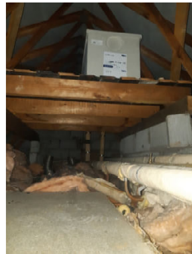
Photograph 4: Loft void in the Eastern wing of building 1.
