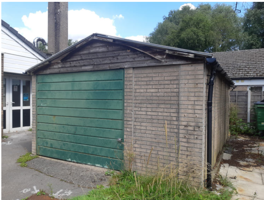
Photograph 1: Building 2; small garage adjacent to main building (building 1).
