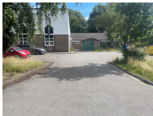
Photograph 6: Parcel of u1b-1, developed land, sealed surface
