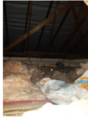
Photograph 8: Loft void in the Southern wing of building 1.
