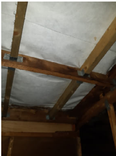
Photograph 3: Loft void in the Northern wing of building 1.
