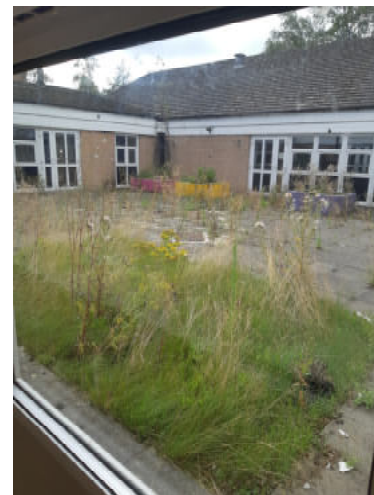
Photograph 12: Central courtyard of building 1 (only visible from the interior of building).
