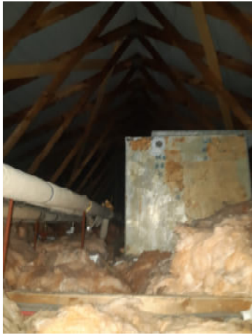
Photograph 1: Loft void in the Northern wing of building 1.
