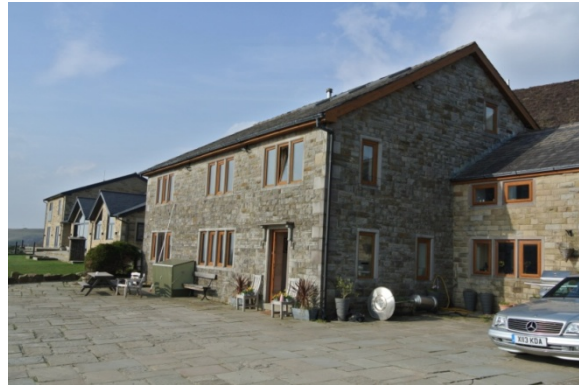
Taller building and barn viewed from the south.
