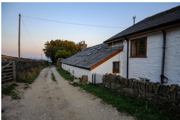
North elevation with mixed random and coursed walling.
