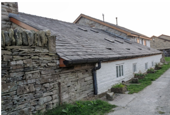
Elevation with catslide roof and watershot wall.
