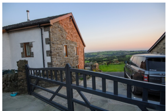
Gable in recent random stonework.
