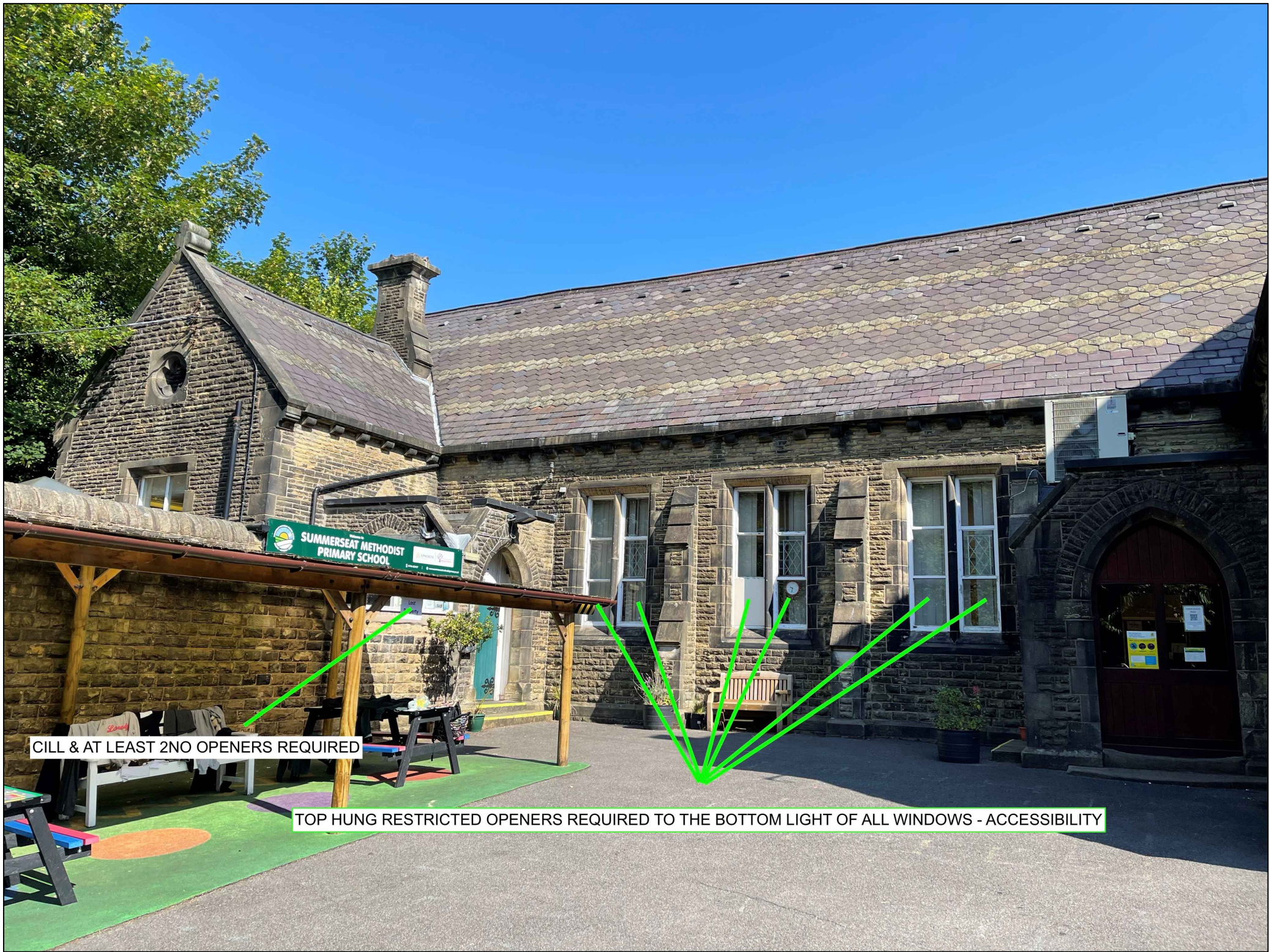
Summerseat Primary School - Window Elevations - Images NTS
