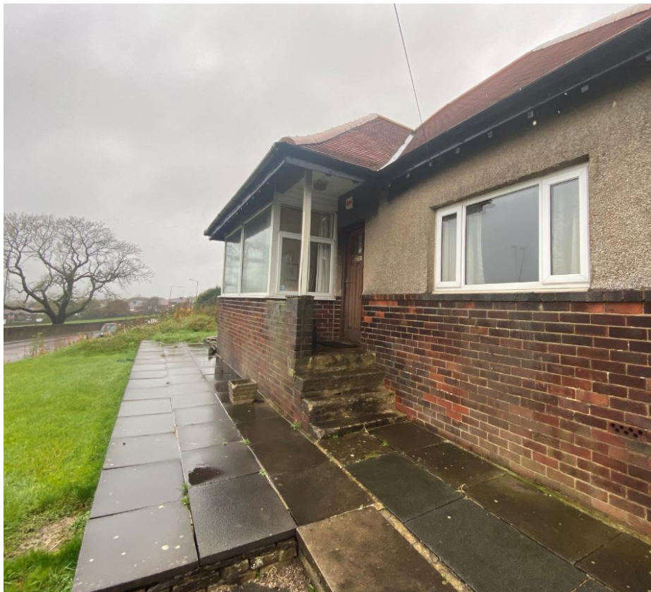
Photograph of Existing open porch area
