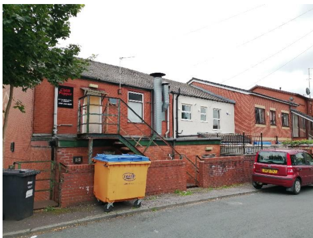
Figure 5.1: Rear elevation of commercial units viewed from Quarry Street.
