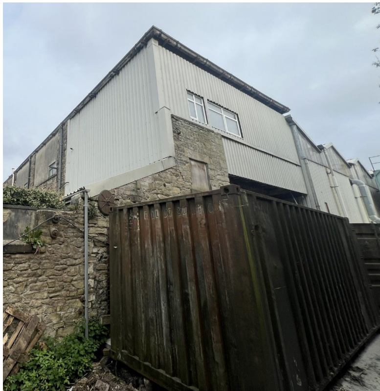
Figure 10 | Existing storage porta cabin
