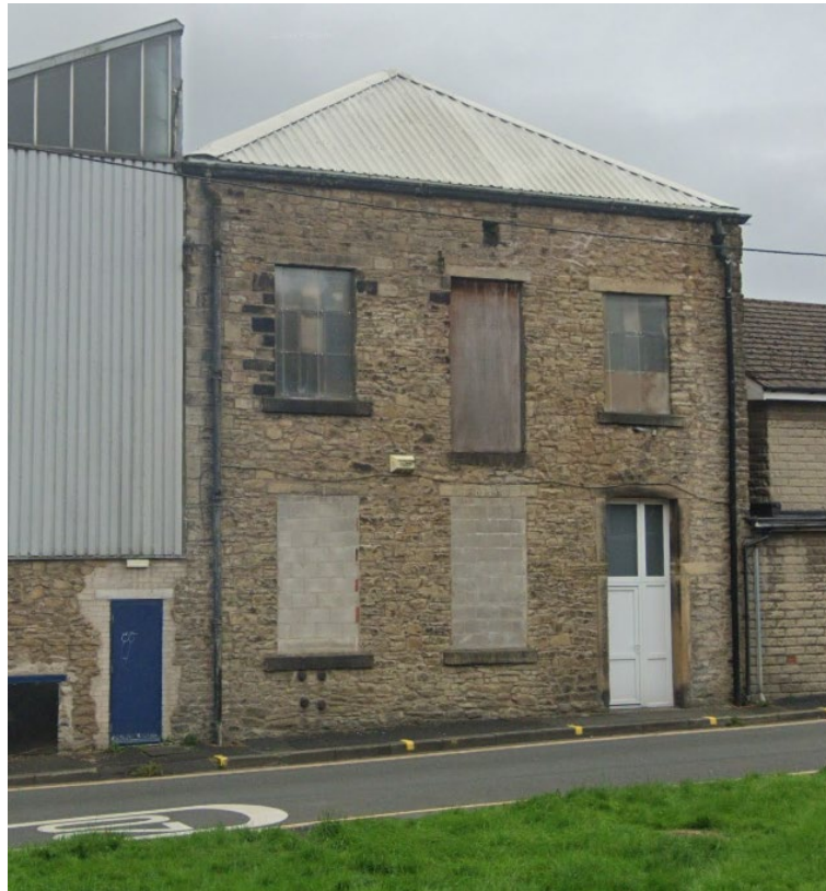
Figure 5 | Image of natural stone factory building | Google Images | not to scale
