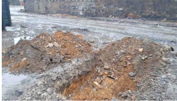
Trial Pit 5 Arisings
