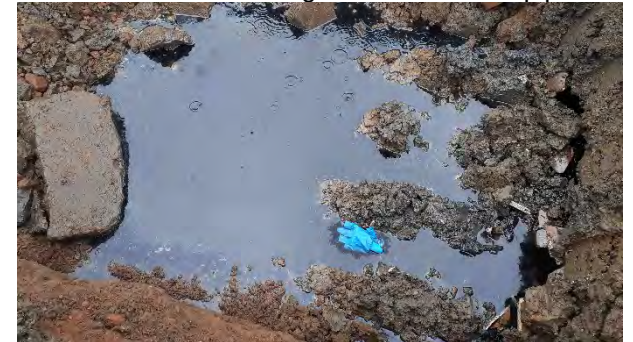
Trial Pit 4 - Water ingress from broken pipe
