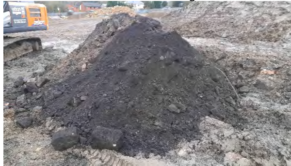
Trial Pit 2 Arisings
