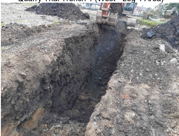
Quarry Trial Trench 1 (West - Log 4 Area)
