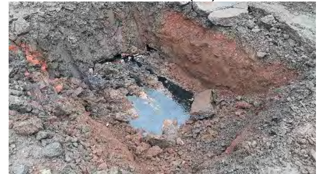
Trial Pit 4 - Water ingress from broken pipe
