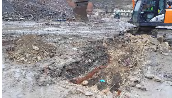
Trial Pit 2 Arisings
