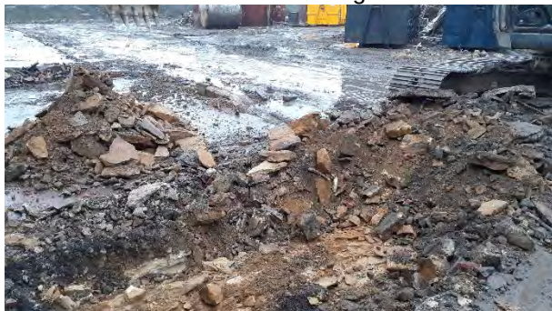
Trial Pit 1 Arisings
