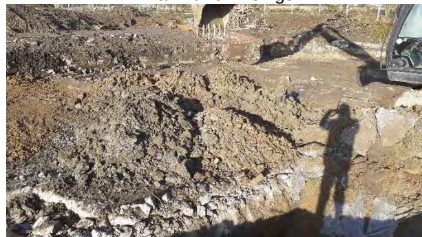
Trial Pit 10 Arisings
