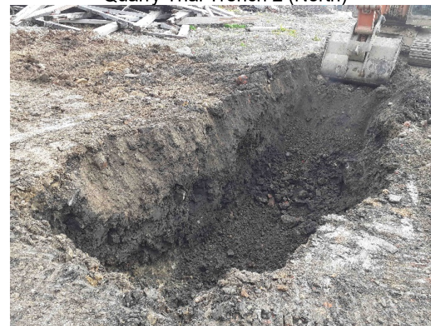
Quarry Trial Trench 2 (North)
