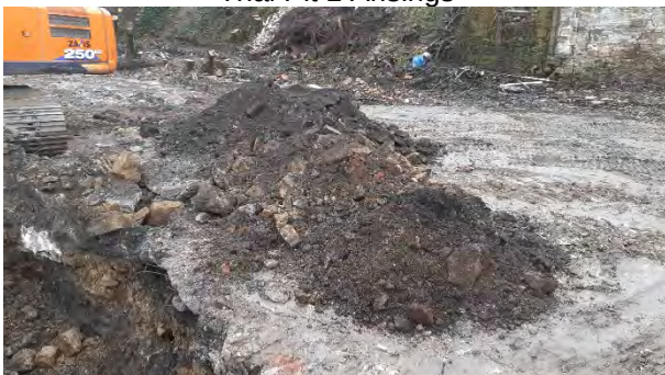
Trial Pit 1 Arisings
