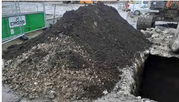
Trial Pit 2 Arisings
