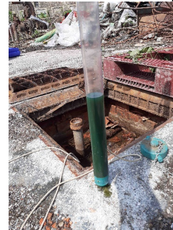
Inspection Chamber 10 Sample
