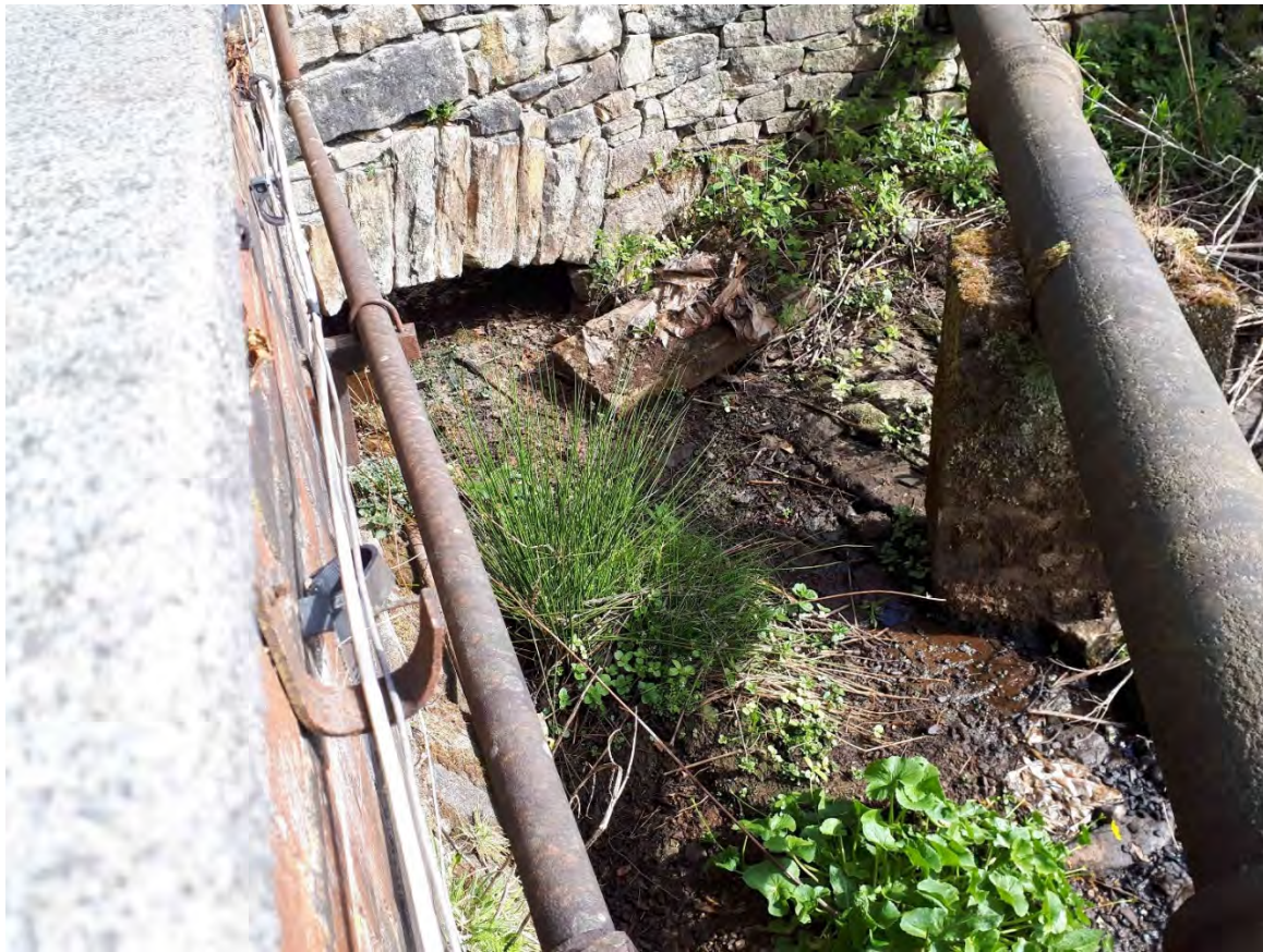
Historical feature northern area of Phase 2
