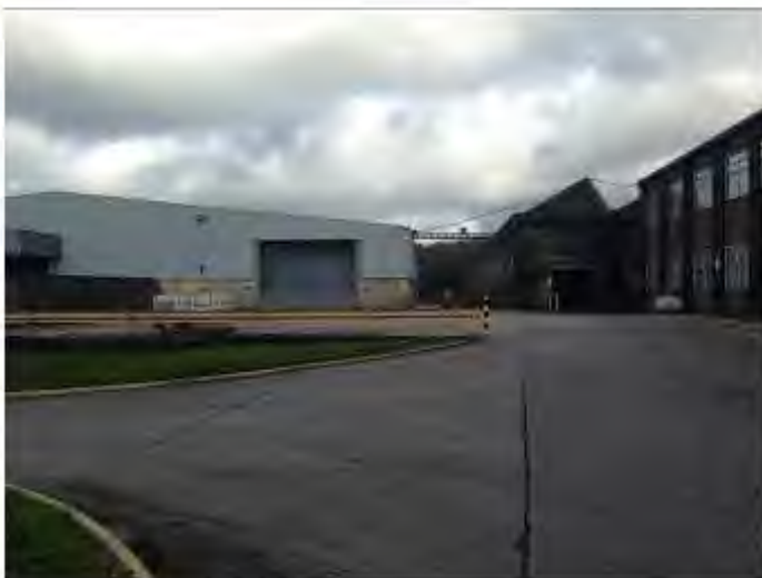
Plate 3 – Portal Frame Distribution Shed in North West Sector
