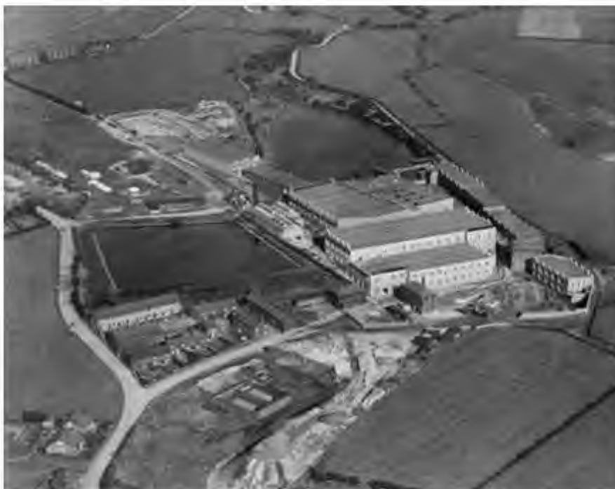
Figure 3.1 gives an overview of the site with two large reservoirs to the north and west and main mil complex to the central and southeast. The landform has been dammed to allow the collection of water with mill buildings having been built into the hillside to create a split level site.
