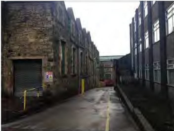
Plate 1 – Mill Buildings through central sector of the site
