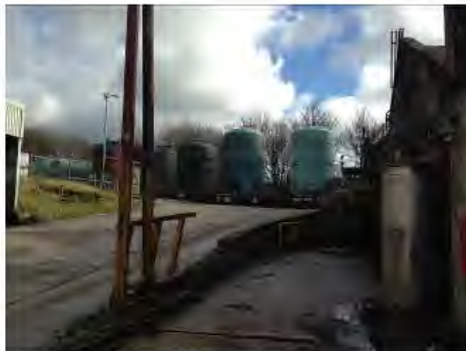
Plate 15 – Wider View of Tank farm to North
