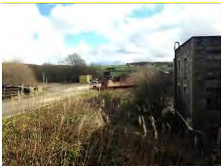
Plate 5 – Reservoir Dam Looking East
