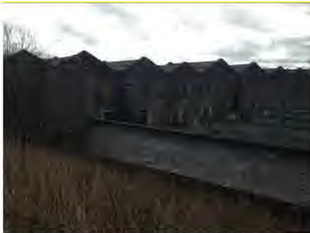
Plate 7 – Dam Looking Southeast Showing Split Level Site
