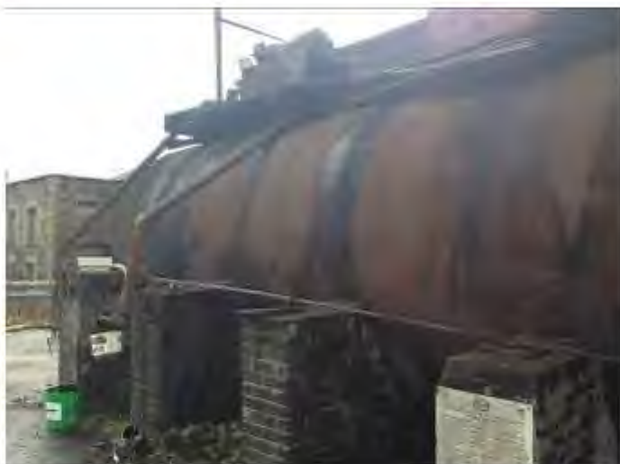
Plate 4 – Bitumen Tank on Reservoir Dam
