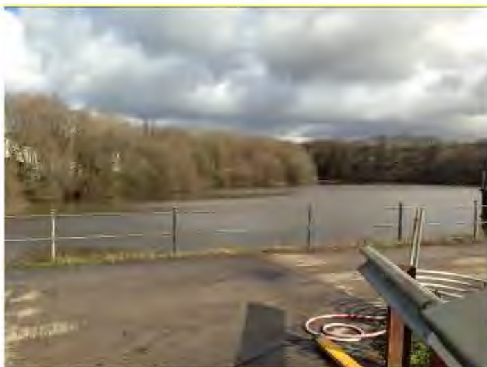
Plate 6 – Reservoir Looking North
