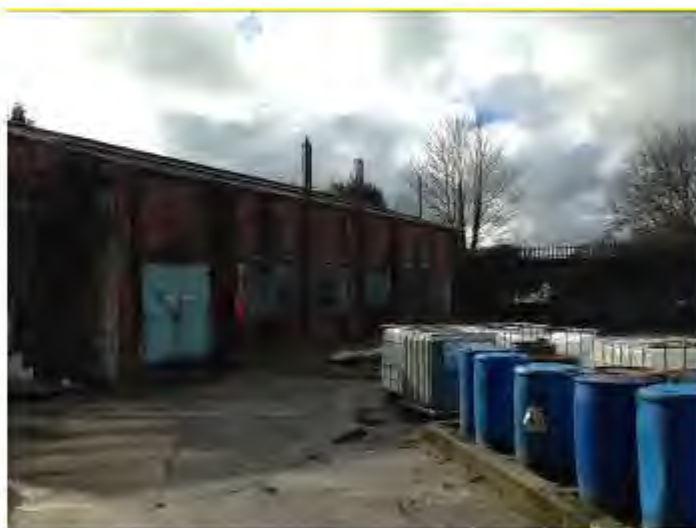
Plate 12 - Far Southern sector showing Underground Tank Farm and Ventilation Pipes
