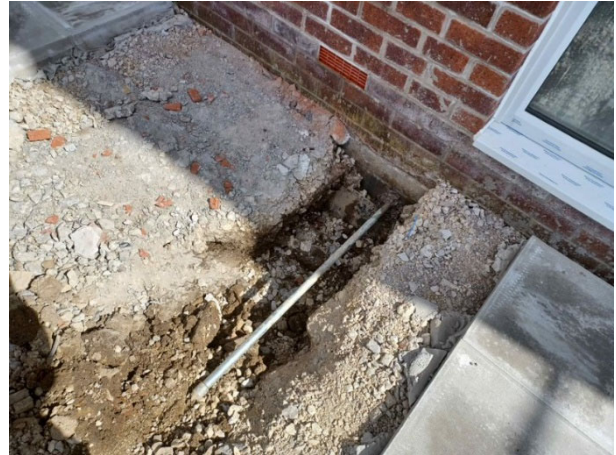
Plot 63 (VP1) sub-floor void installation
