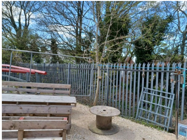
Control (VP4) installation location
