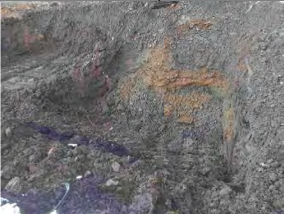
Second dig in north side (south backfilled with clen overburden)
