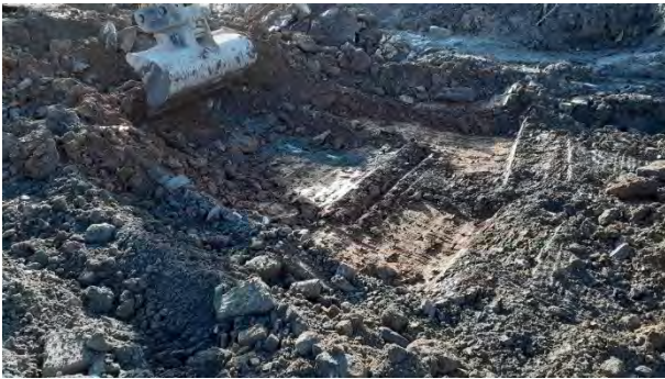
Photograph 35 – Southern extent of excavation
