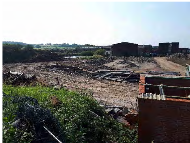
Photograph 10 – Southern section of site from northern Phase 2A
