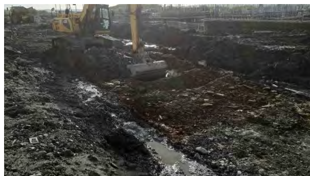
Photograph 32 – Excavation at centre of cell
