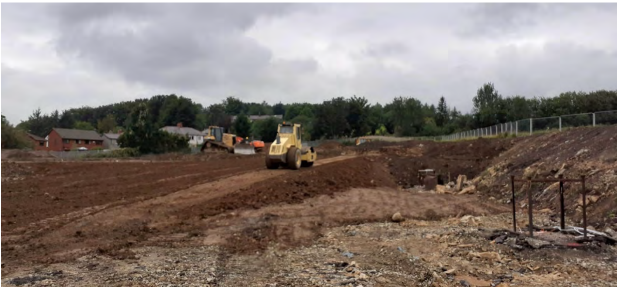
Photograph 11 – Upfilling of site levels at Phase 1/Phase 2A boundary
