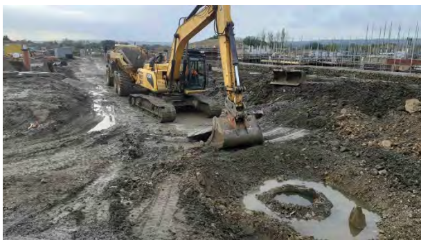
Photograph 29 – Removal of concrete road (0.2m bgl) to north
