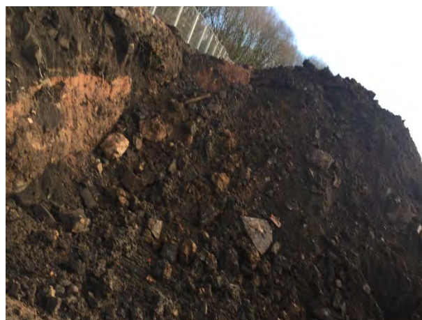
Photograph 21 – Proof dig of upper fills in quarry north Phase 2A
