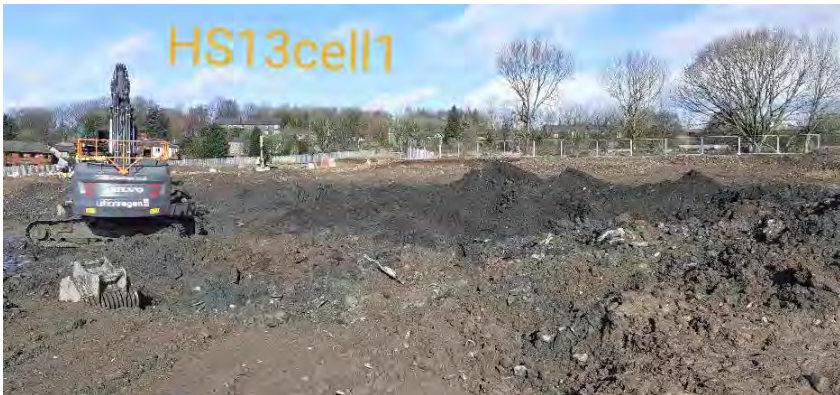
General view after excavation
