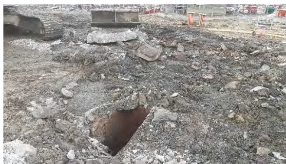
Photograph 26 – Manhole chamber in Phase 2A.
