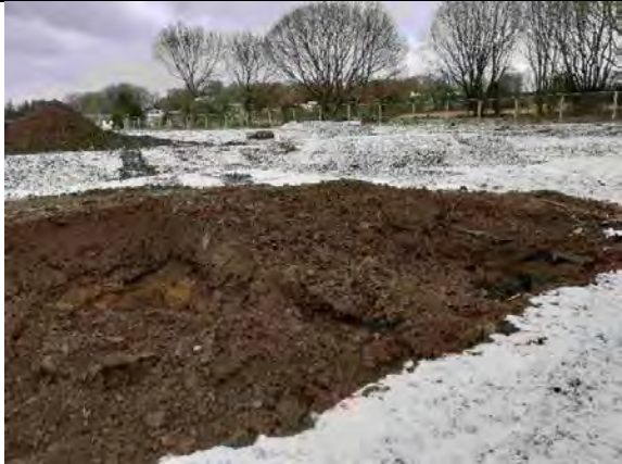
Extent of excavation
