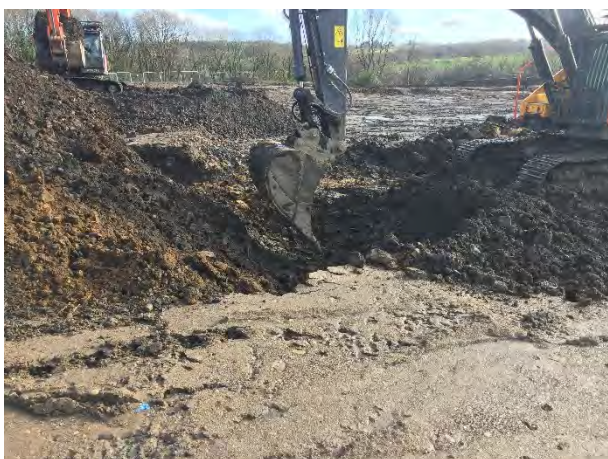
Photograph 22 – Proof dig of upper fills in quarry north Phase 2A
