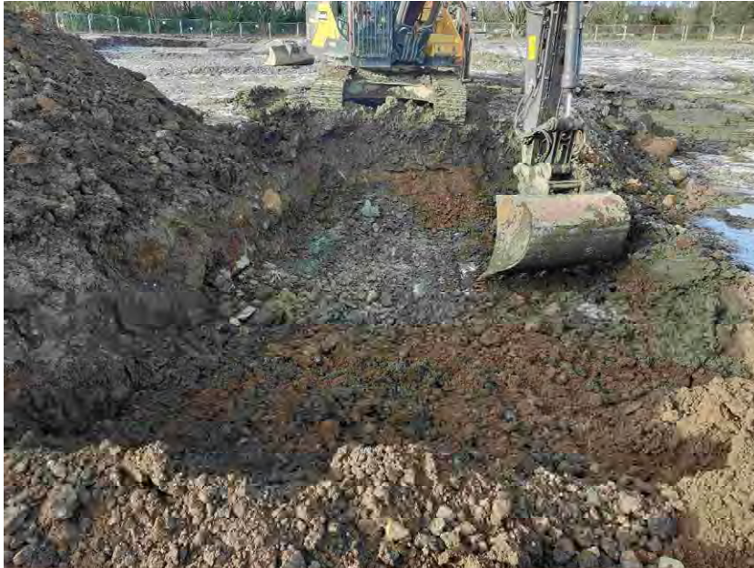
General view north over Cell
