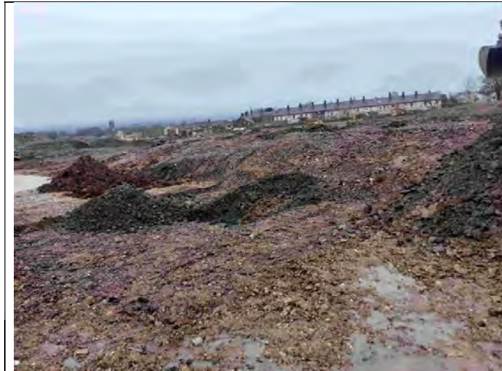
Initial Trial Pits Excavated to locate start remediation excavation and establish depth
