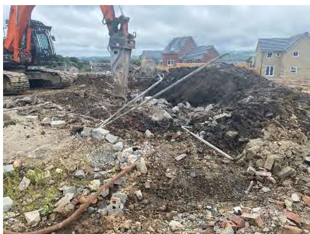
Photograph 37 – Breaking out concrete substructure surrounding tanks
