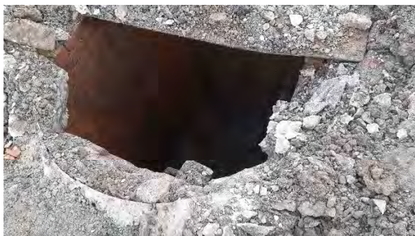
Photograph 27 – Manhole chamber in Phase 2A.
