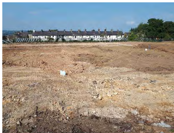
Photograph 8 – Centre of Phase 1 from Phase 2A
