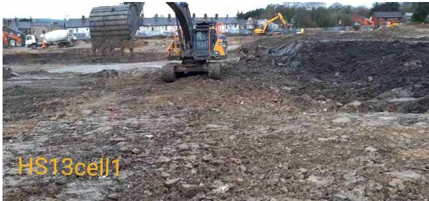
General view before excavation
