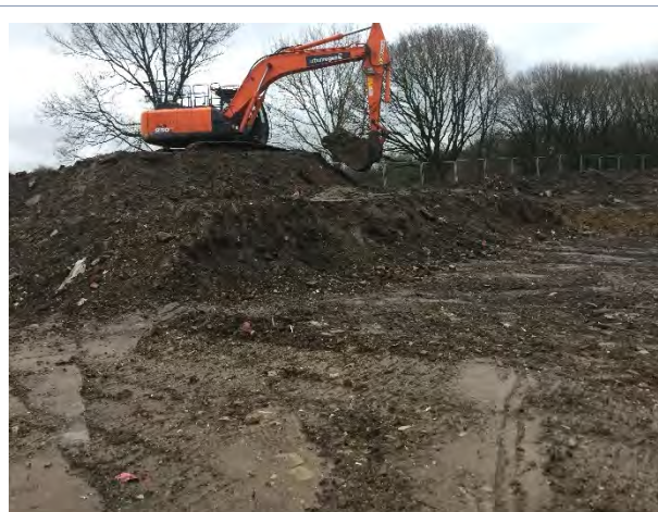
Photograph 19 – Reduced level dig of former quarry (Phase 2A)
