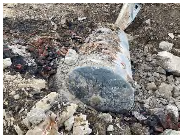
Photograph 39 – Removal of substructure at tanks
