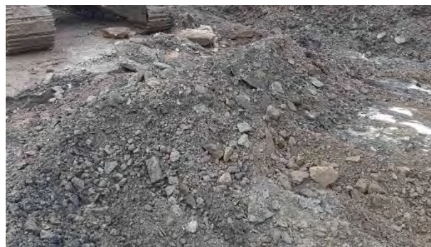
Photograph 30 – Arisings from northern excavation
