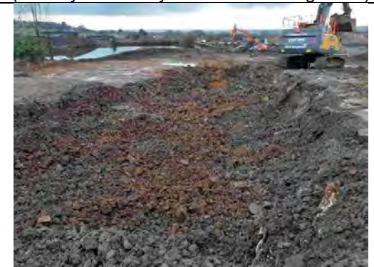
Cell backfilled with clean overburden and recycled aggregate
