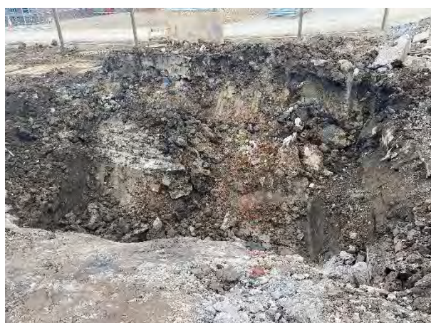
Photograph 40 – Made Ground soils following removal of tank
