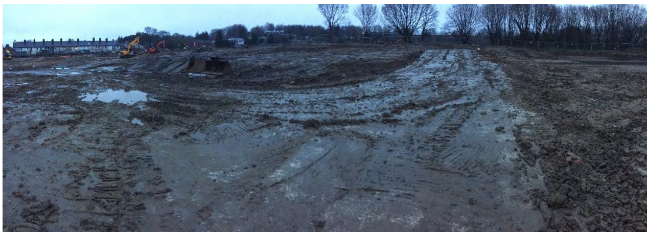
Photograph 24 – Completion of the northern Phase 2A area following reduced level dig and proof dig to former quarry
