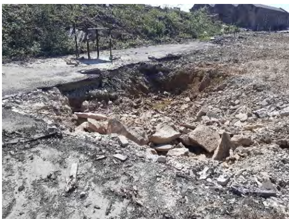
Photograph 1 – North eastern corner of northern building in Phase 2A.
