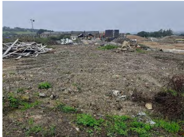
Photograph 13 – Former roadway at Phase 2A (right) from quarry area
