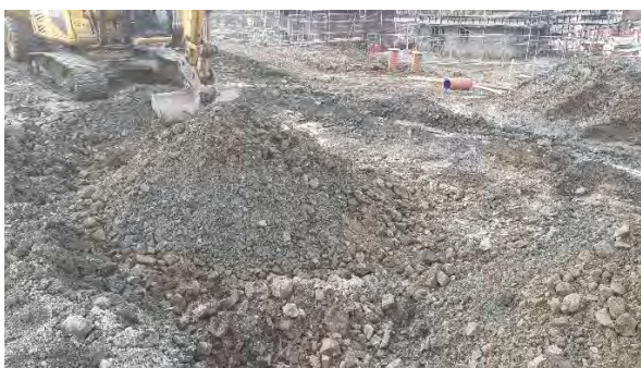
Photograph 25 – Stockpile of granular MG south of HS10 (Cell 6)
