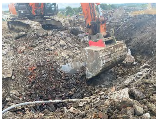
Photograph 38 – Excavation of substructure/MG soils at tanks
