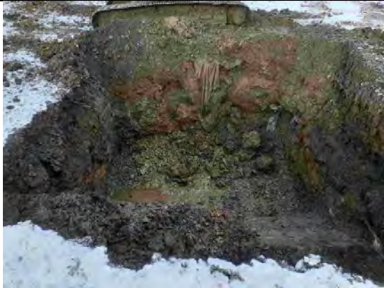
Initial dig in south side
