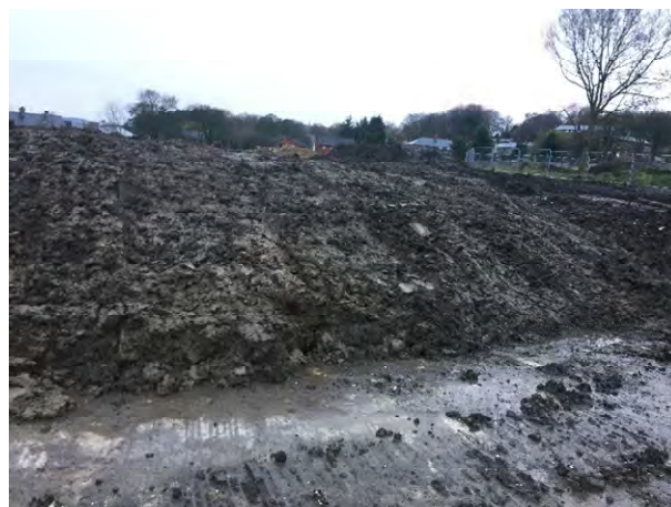
Photograph 17 – Reduced level dig of former quarry north Phase 2A
