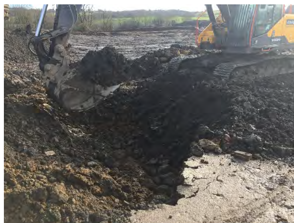
Photograph 23 – Proof dig of upper fills in quarry north Phase 2A
