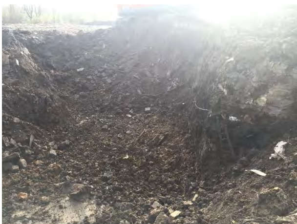
Photograph 20 – Proof dig of upper fills in quarry north Phase 2A
