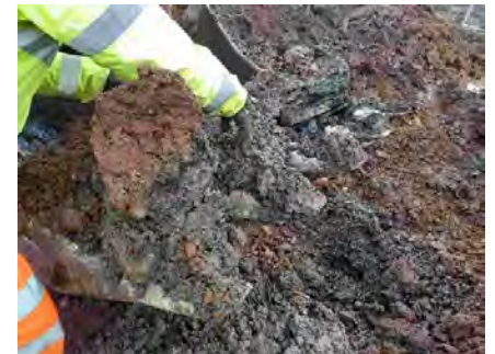
Boundary between natural clay (excavated) and underlying Rough Rock (excavated to competent rockhead)
