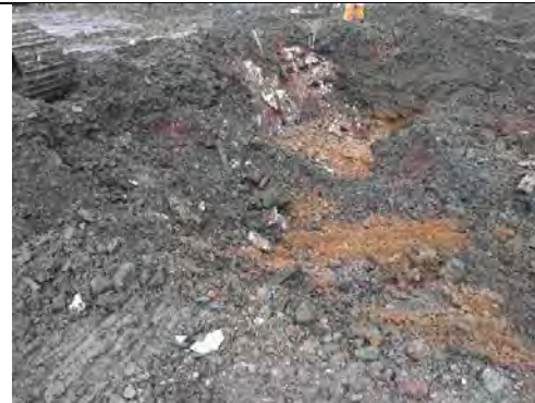
Excavation extended through granular made ground
