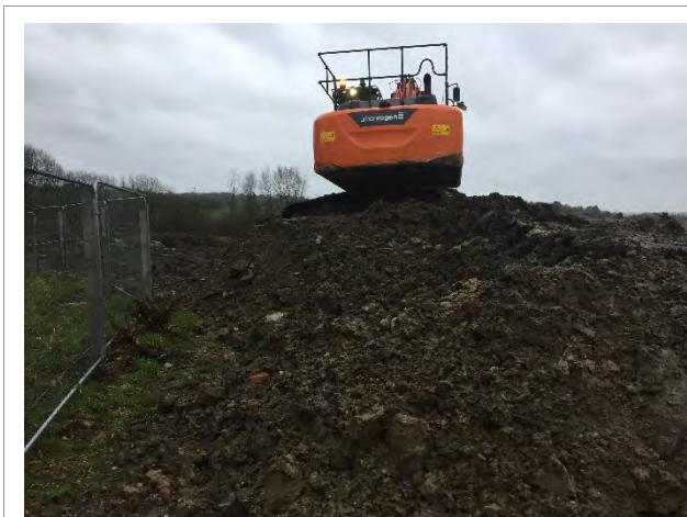
Photograph 18 – Reduced level dig of former quarry (Phase 2A)
