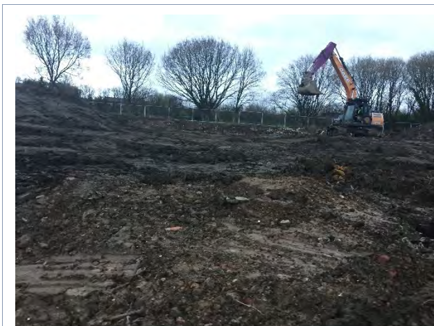
Photograph 16 – Reduced level dig of former quarry north Phase 2A
