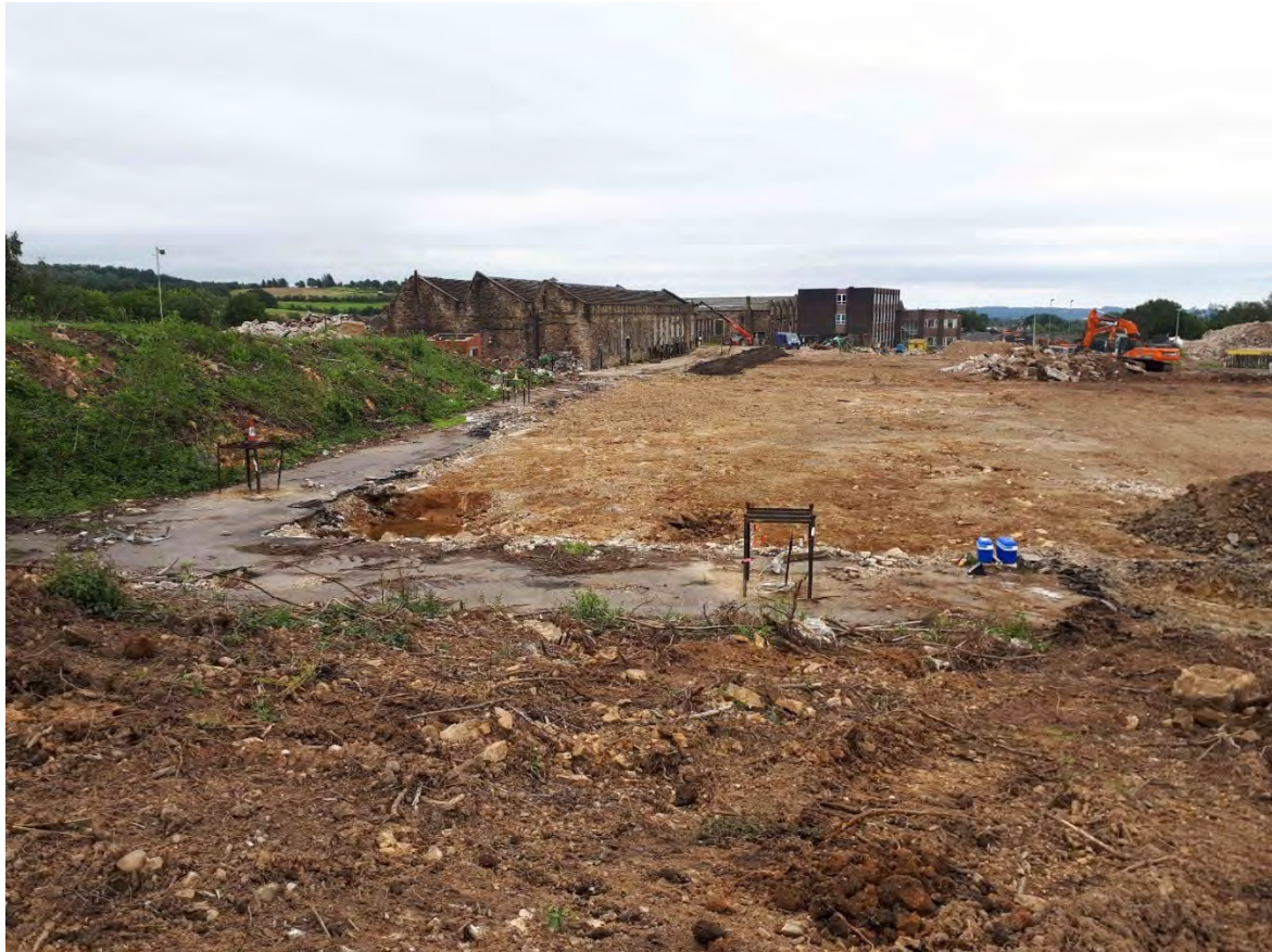
Photograph 5 – Northern end of Phase 1 (right) & Phase 2A (left)
