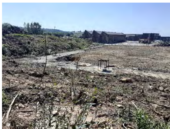
Photograph 4 – Former building in northern area of Phase 1
