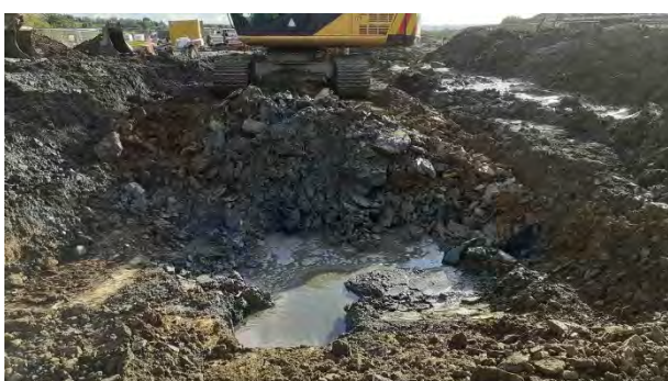
Photograph 33 – Southwards excavation progression
