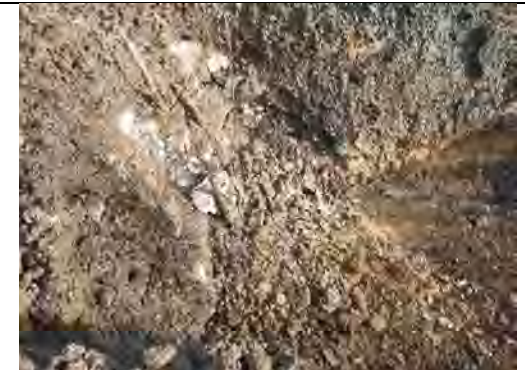
Excavation extended to competent rough rock where contamination indicators present (mainly below clay in weathered rough rock)
