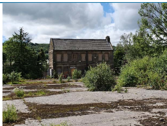
Photograph 1: Eastern elevation of building B1
