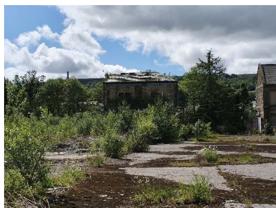
Photograph 2: Eastern elevation of Building B2
