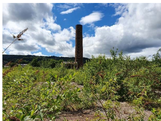
Photograph 3: Eastern elevation of building B3 and chimney
