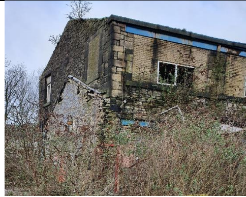
B2, demolished section to the southern elevation
