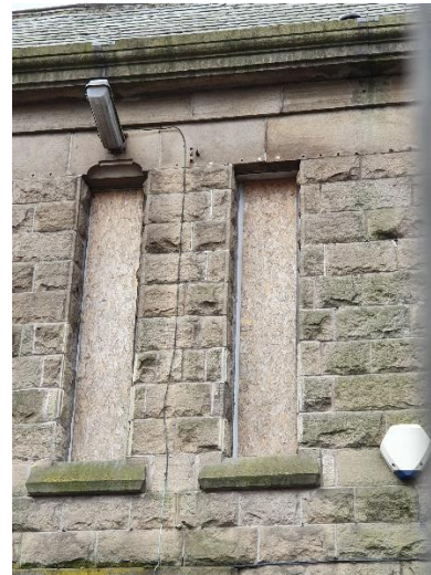
B1 Visible gaps beneath stone window ledge
