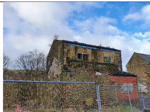
B2 eastern elevation with single storey extension
