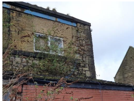
B2 Supporting beam to the eastern elevation
