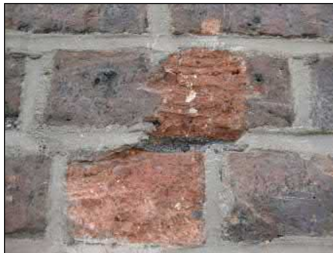
Indication of previous repointing
