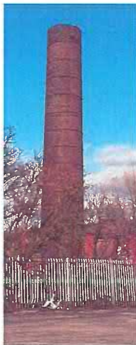
Picture 1 – General view of chimney
