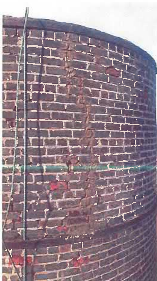
Picture 3 – Crack repairs to southern elevation
