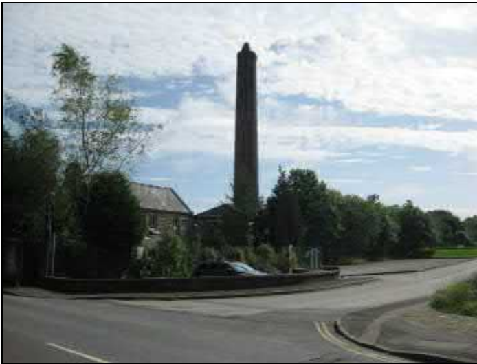
Elevation from NW showing lean to South West
