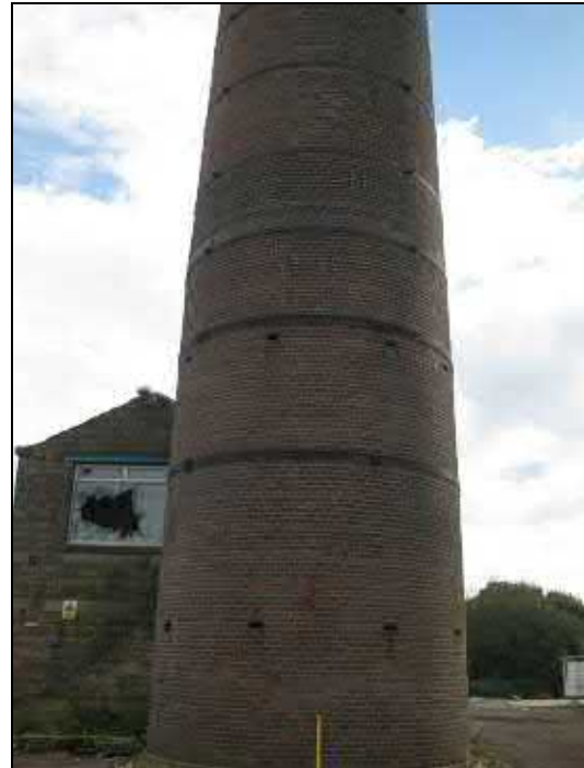
North elevation showing previous repair at approximately 10m
