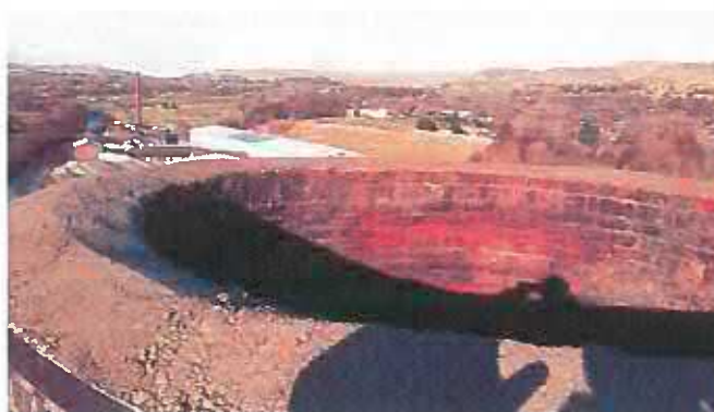
Picture 2 – Vie of concrete Haunch
