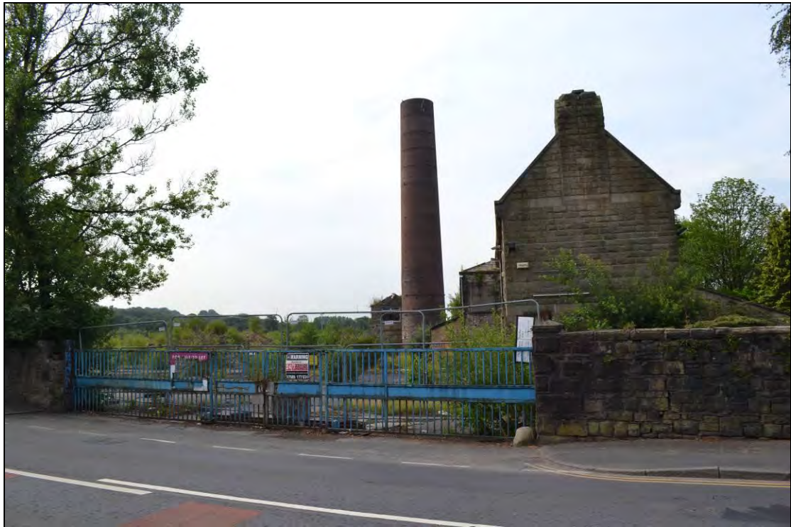
Photograph 43: View south of site from across Bridge Street
