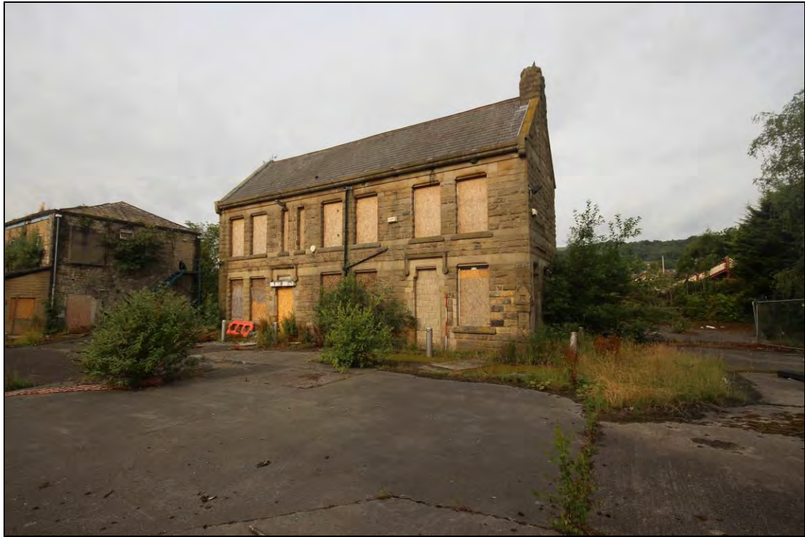
Photograph 23: View of building A and the architectural detailing, facing south-west, 2m scale
