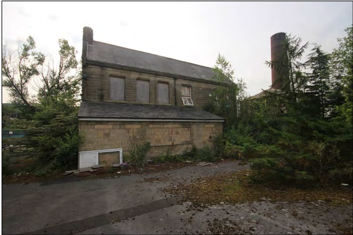
Photograph 25: View of the western elevation of building A with the lean-to extension, 2m scale
