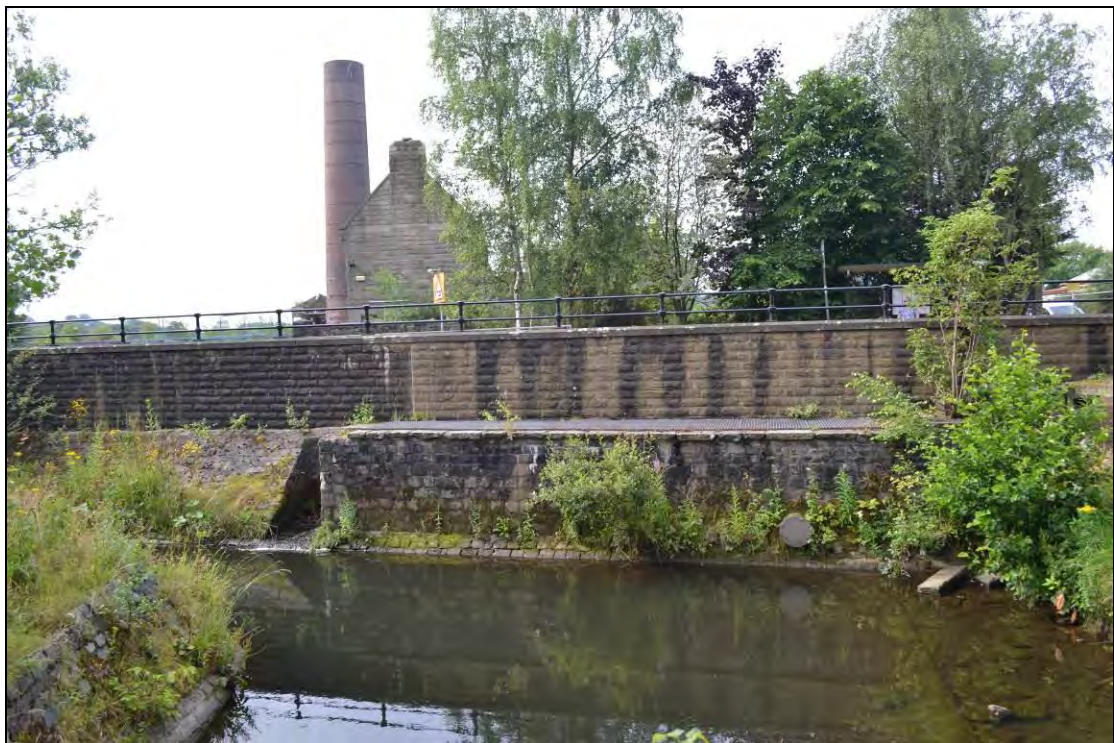
Photograph 44: View south from within park
