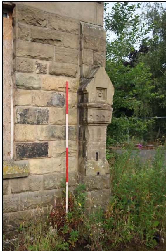
Photograph 22: View of a potential gatepier along building A, 2m scale
