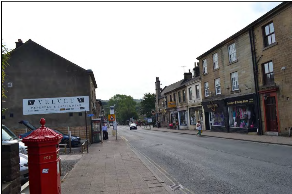
Photograph 40: View east along Bridge Street
