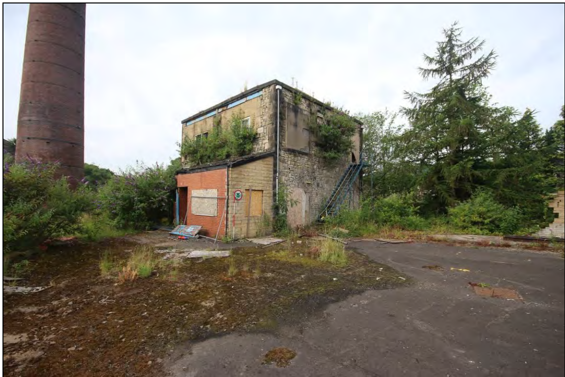
Photograph 26: View of building B, facing south-west, 2m scale
