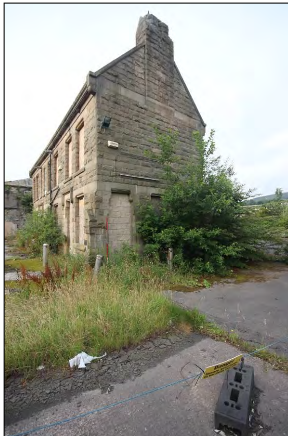
Photograph 24: View of the northern gable end of building A, 2m scale
