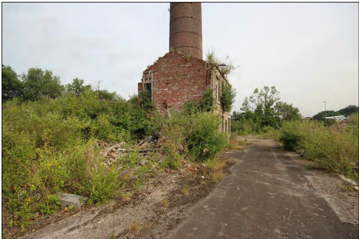
Photograph 30: General view of building C, facing north
