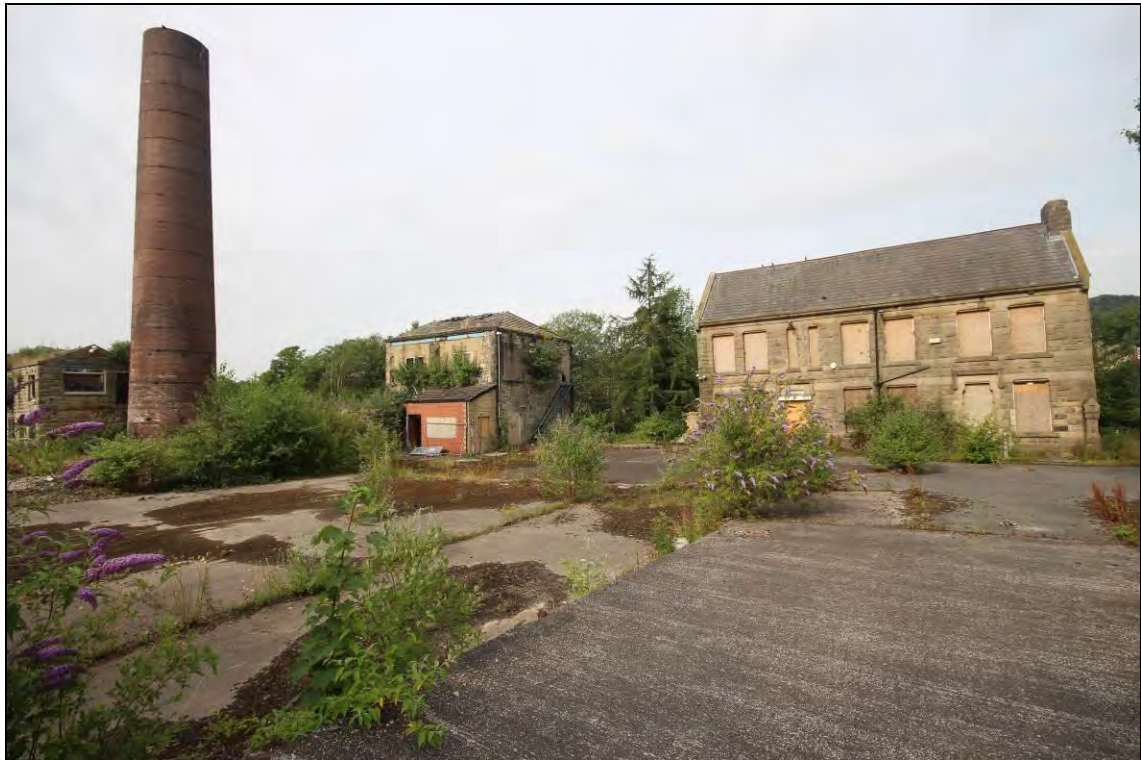
Photograph 19: General view of three buildings and chimney remaining on site, facing south-west
