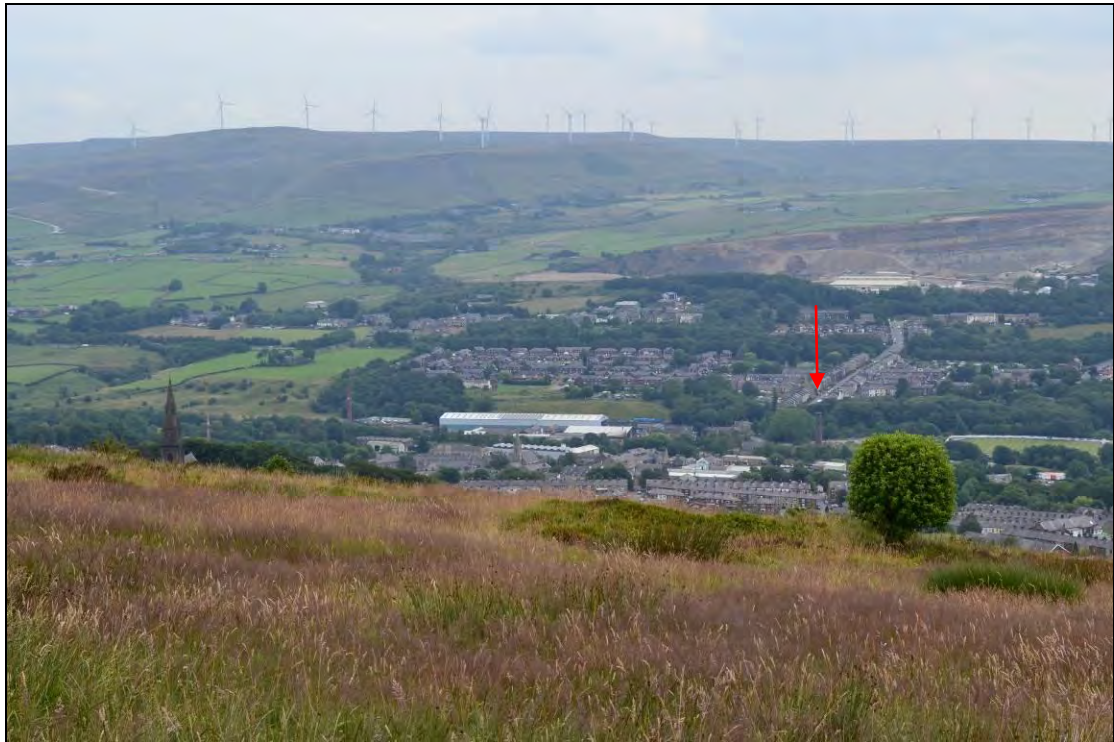
Photograph 35: View north-east from Peel Tower across Ramsbottom. Holcombe Mill chimney is indicated by the red arrow
