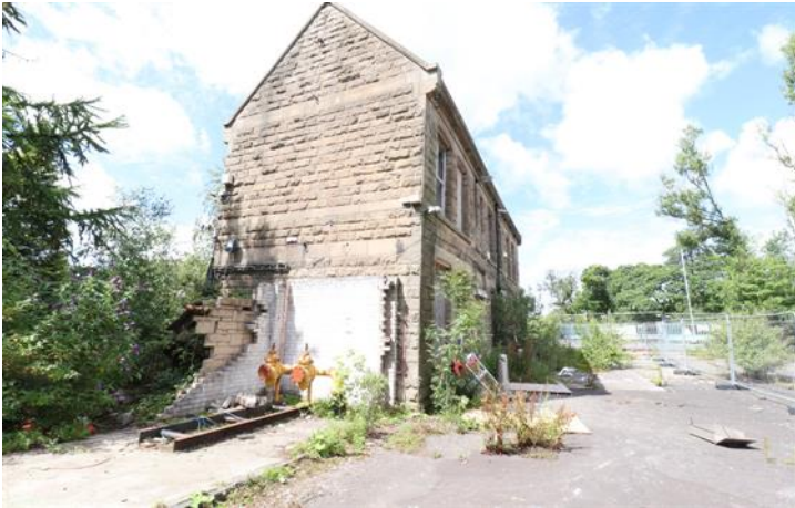
Image 3 – Existing Building A, South Elevation
