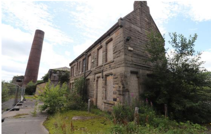
Image 6 – Existing Building A, North and East Elevations
