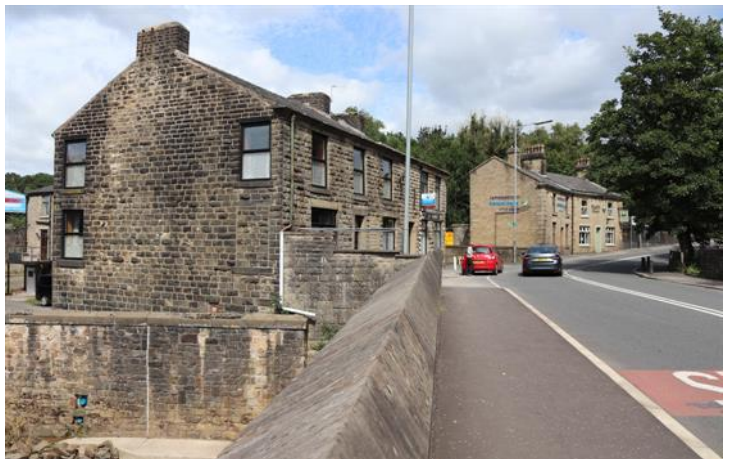
Image 24 – North-West Facing Views from Bridge
