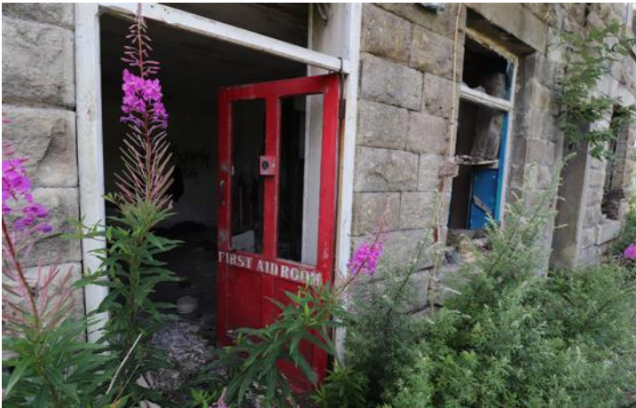
Image 13 – Existing Building B, East Elevation
