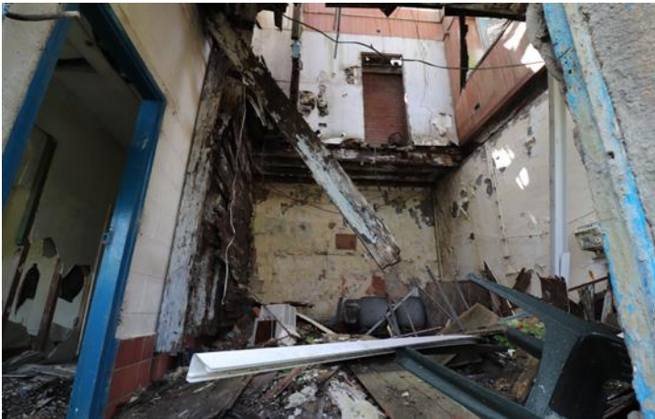
Image 15 – Existing Building C Interior
