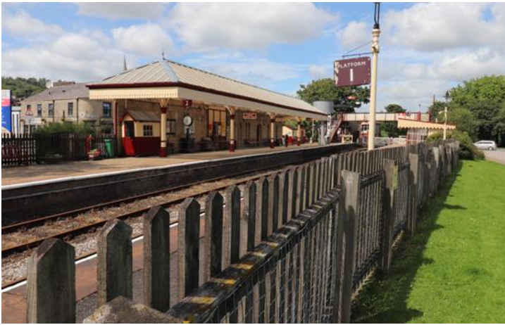
Image 27 – North-West Facing View Of Train Station From Road I
