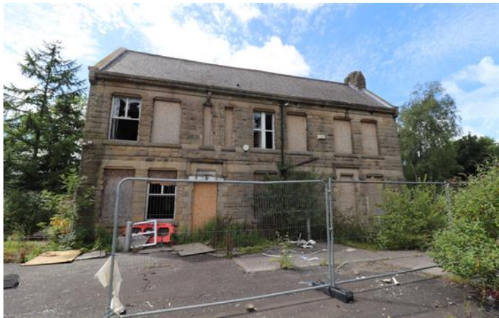
Image 2 – Existing Building A, East Elevation
