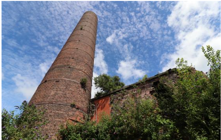
Image 14 – Existing Building C (West Elevation) Plus Chimney
