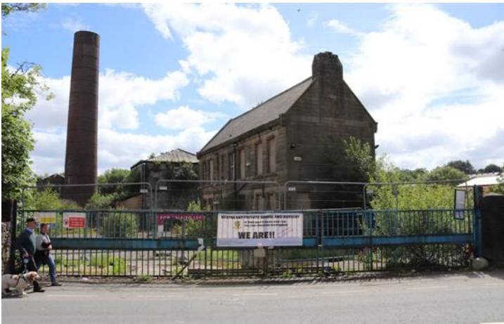
Image 1 – South facing view of site from bridge Street
