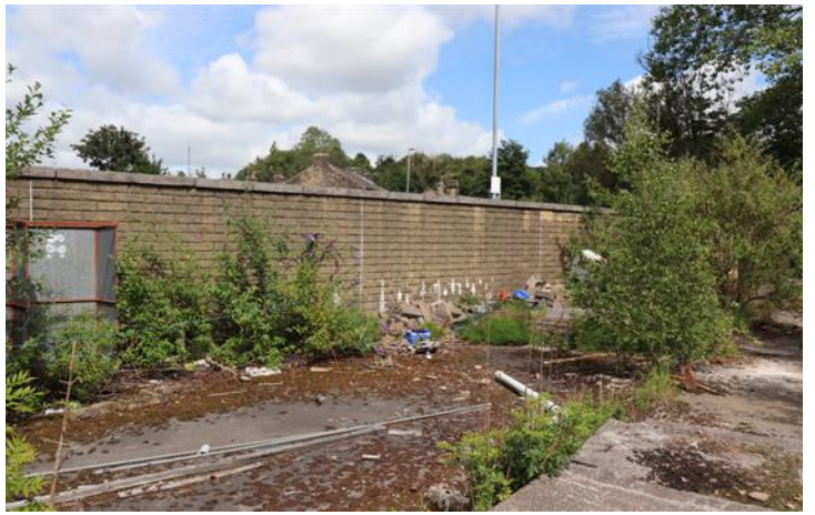
Image 18 – Northern Boundary Of The Site Including Existing Wall
