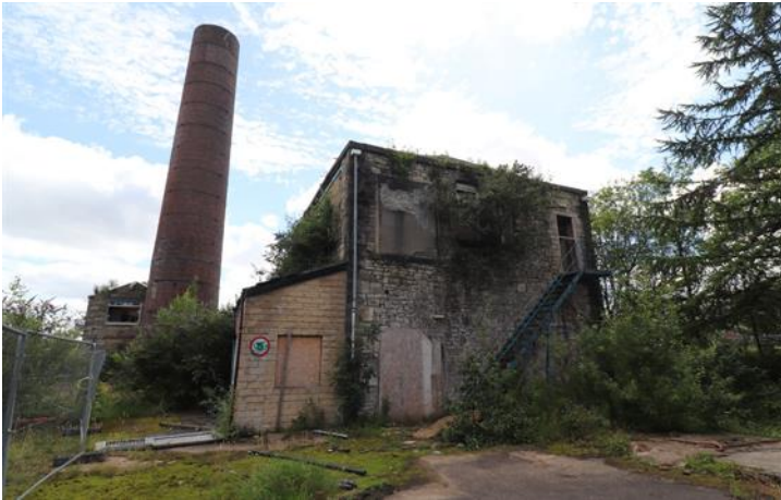
Image 7 – Existing Building B – North Elevation
