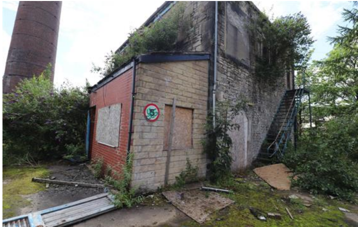
Image 8 – Existing Building B, North and East Elevations
