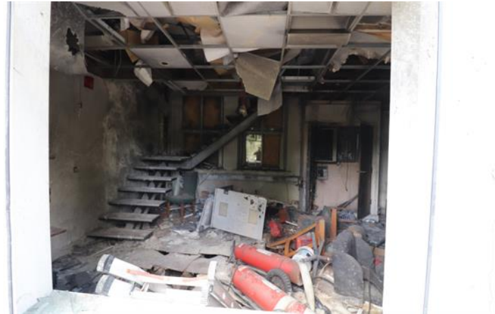
Image 4 – Existing Building A, Interior
