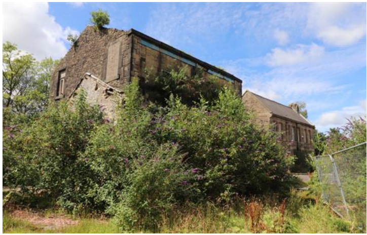
Image 10 – Existing Building B (Foreground) South and East Elevations
