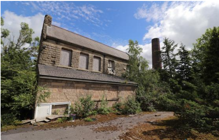
Image 5 – Existing Building A, West Elevation
