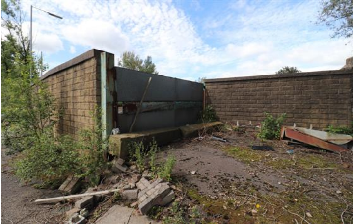
Image 19 – Gate on Northern Boundary Wall at Curve of Bridge Street
