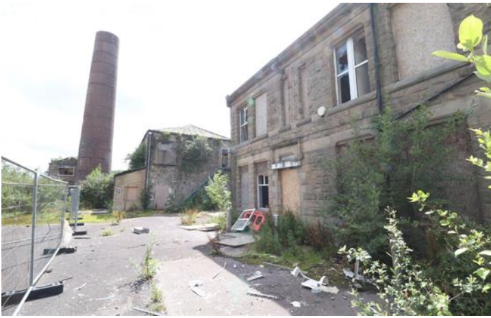
Image 9 – Building A (Foreground) Buildings B and C (Background)
