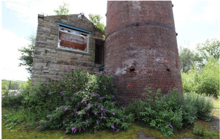
Image 12 – Existing Building C North Elevation (And Chimney)
